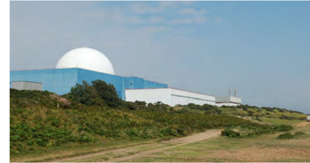
Sizewell power station
