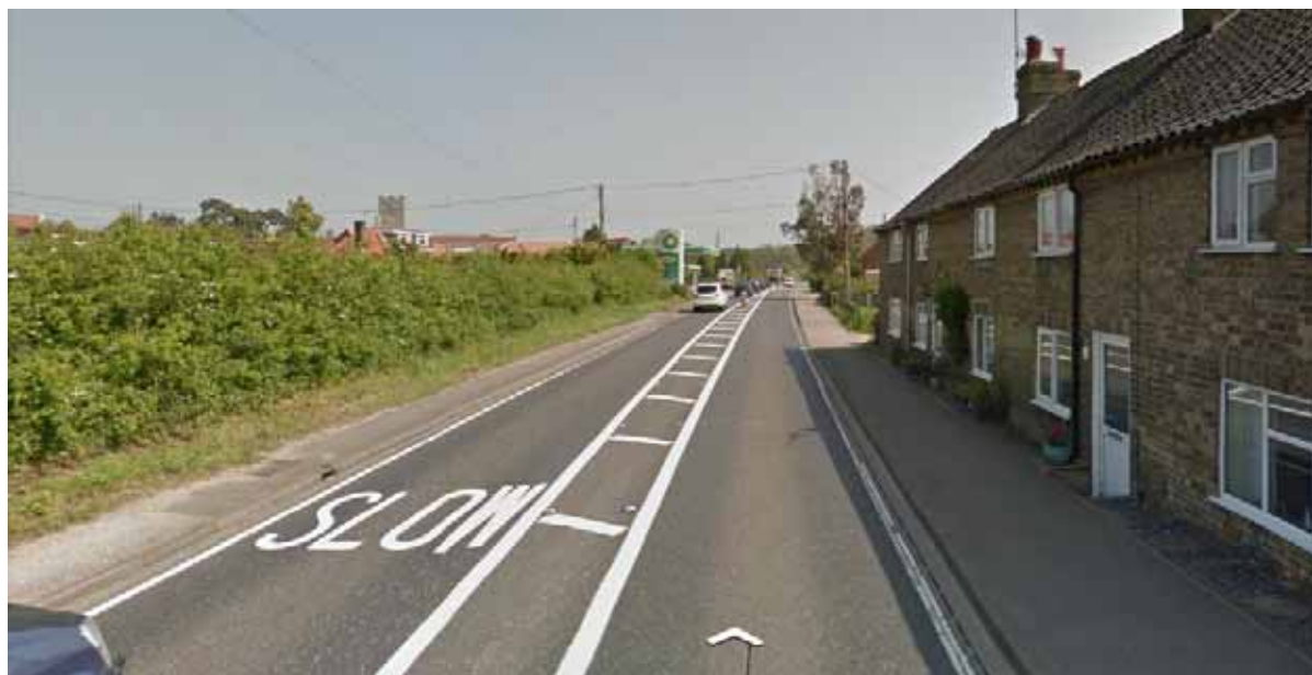
Figure 4: Long row cottages, approaching from the south.
