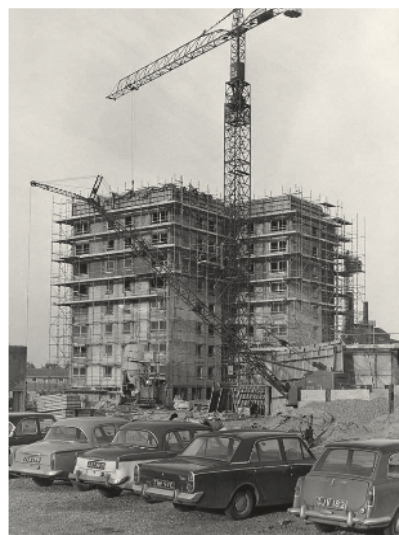
St Peters Court mid construction in 1968
