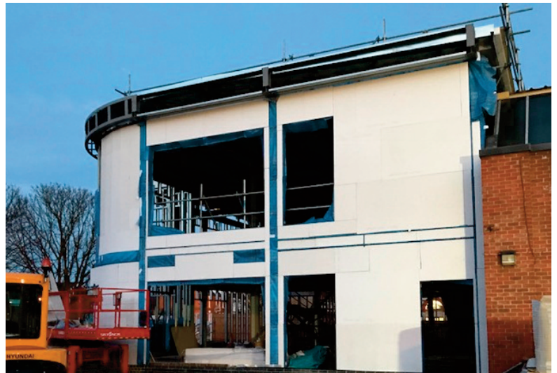
The front to the new leisure facility is almost complete!
