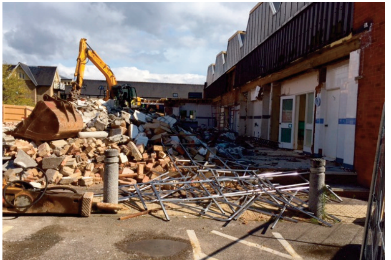
The front of the building was demolished in just a week
