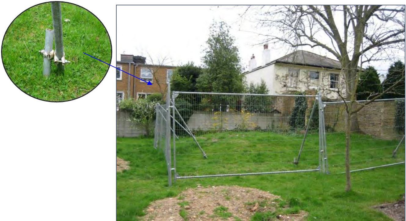
Figure 1 Example of welded mesh barriers in use
