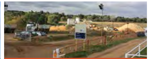
Existing mineral extraction on site
