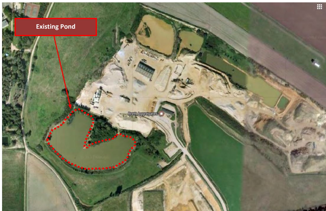
Figure 4a: Existing Pond
