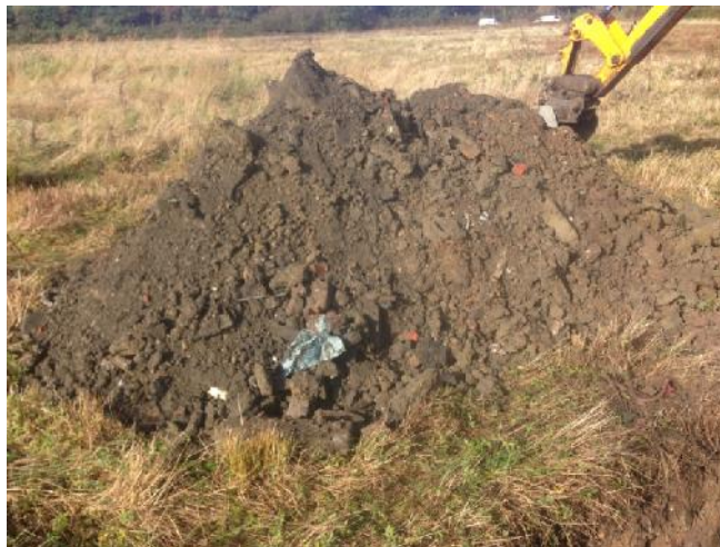
Photo 76: Arisings from trial pit TP23.
