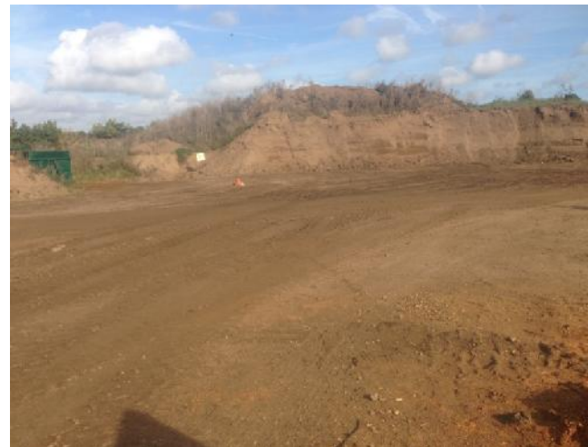
Photo 32: Updated view north of eastern section of Area 1, after spoil had been removed (WS08 now destroyed).
