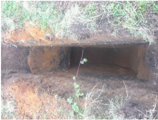
Photo 65: Excavation of trial pit TP17.
