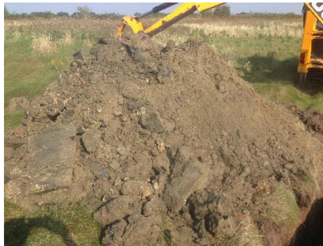
Photo 44: Arisings from trial pit TP06.
