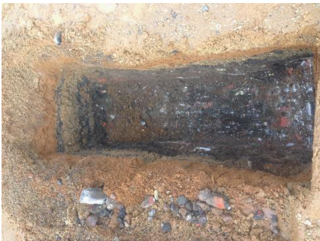
Photo 39: Excavation of trial pit TP04.
