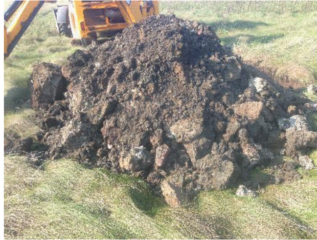
Photo 38: Arisings from trial pit TP03.
