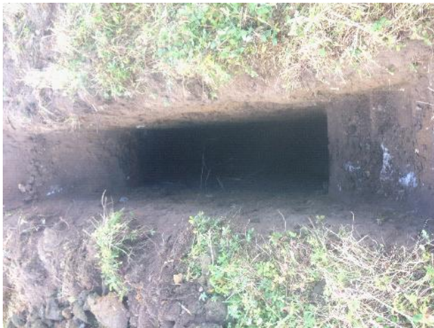
Photo 35: Excavation of trial pit TP02.
