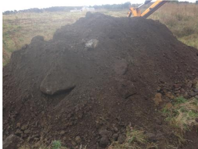
Photo 70: Arisings from trial pit TP20.
