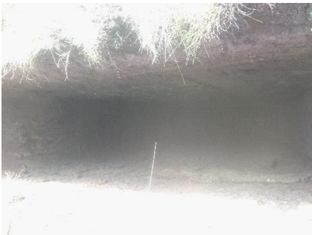
Photo 55: Excavation of trial pit TP12.
