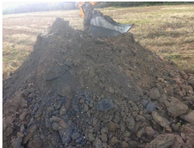
Photo 36: Arisings from trial pit TP02.
