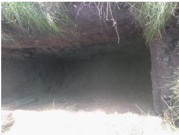
Photo 43: Excavation of trial pit TP06.
