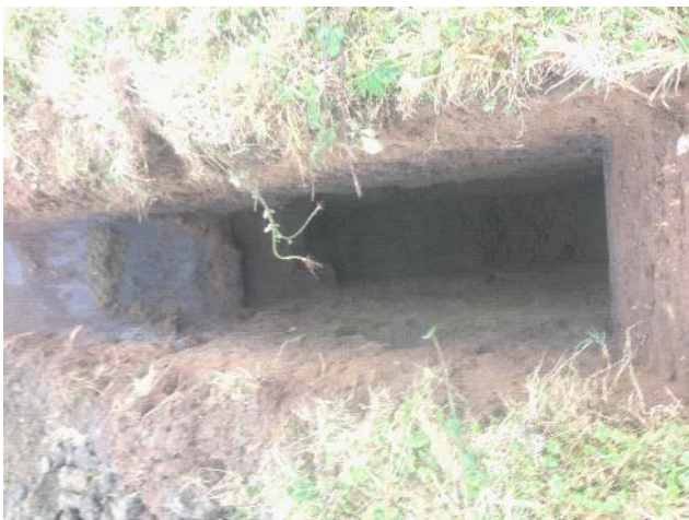
Photo 63: Excavation of trial pit TP16.
