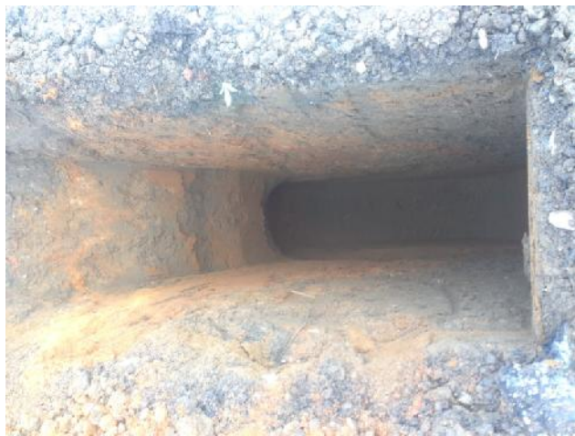
Photo 51: Excavation of trial pit TP10.
