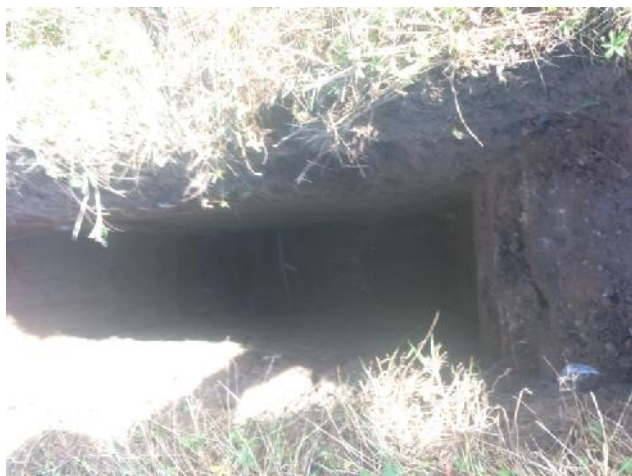
Photo 75: Excavation of trial pit TP23.
