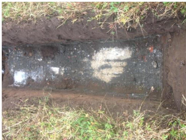
Photo 73: Excavation of trial pit TP22.
