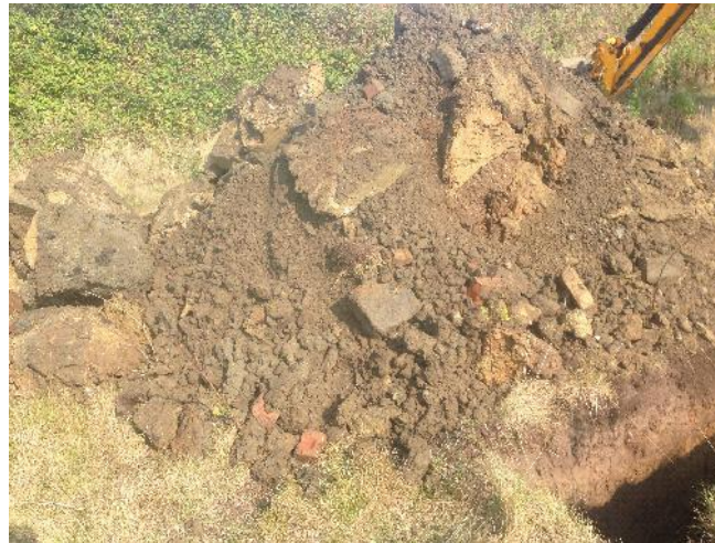
Photo 56: Arisings from trial pit TP12.
