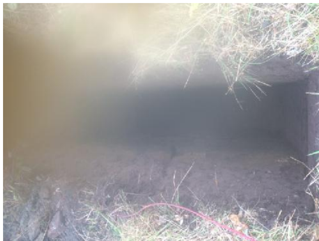
Photo 71: Excavation of trial pit TP21.
