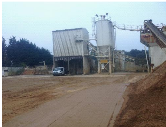
Photo 20: View of concrete mixing plant on the north western corner of Area 1.
