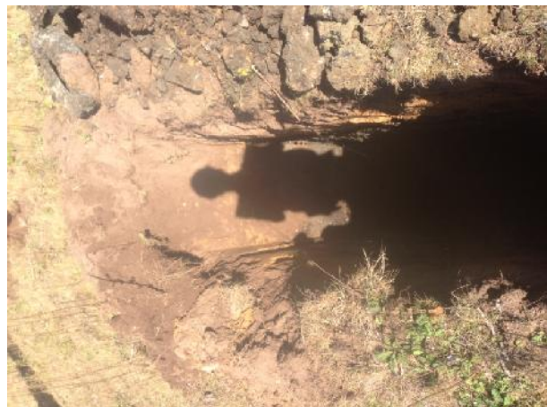
Photo 47: Excavation of trial pit TP08.
