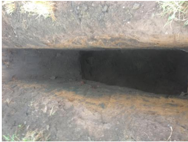
Photo 69: Excavation of trial pit TP20.
