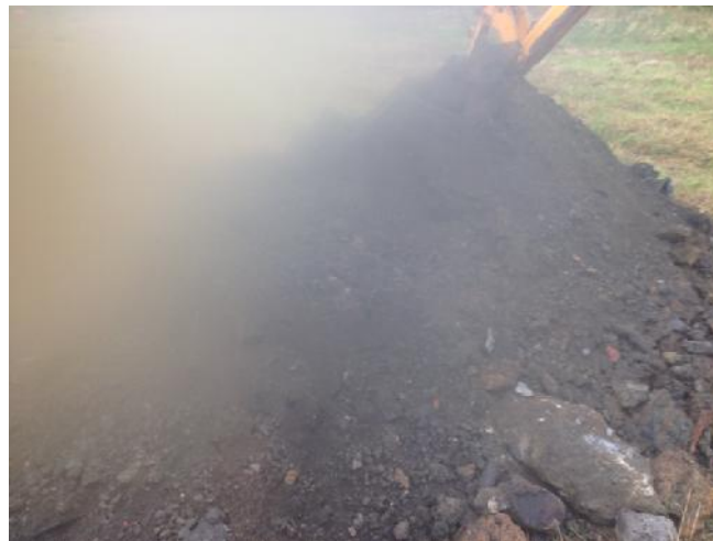
Photo 72: Arisings from trial pit TP21.
