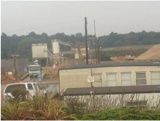
Photo 1: View north of site office in the foreground, weighbridge in the middle ground, and concrete plant in the back ground. (Area 1)
