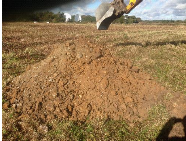
Photo 34: Arisings from trial pit TP01.
