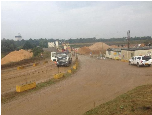
Photo 5: View north west of site office and weighbridge. (Area 1)
