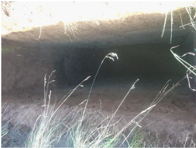
Photo 57: Excavation of trial pit TP13.
