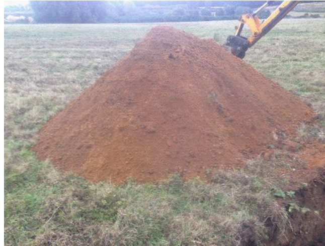
Photo 66: Arisings from trial pit TP17.
