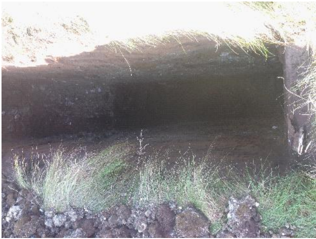
Photo 37: Excavation of trial pit TP03.
