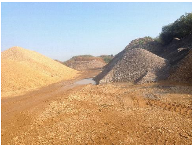
Photo 19: View of mineral storage heaps in central section of Area 1.
