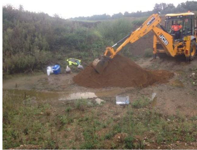
Photo 50: Arisings from trial pit TP09.
