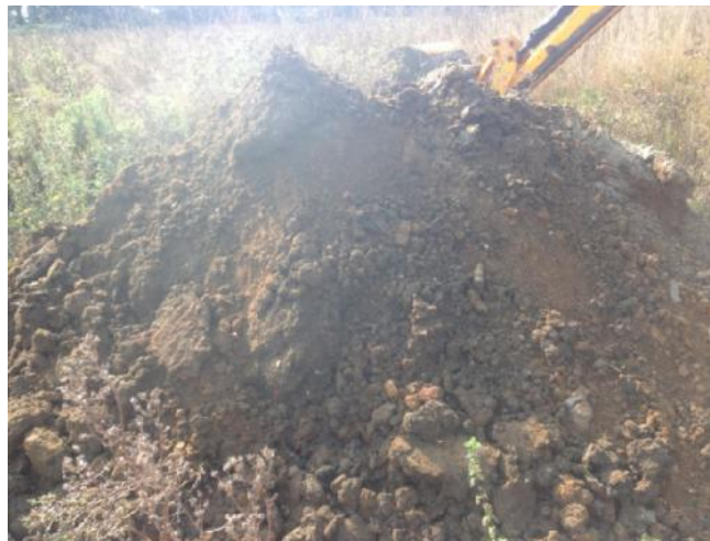
Photo 46: Arisings from trial pit TP07.
