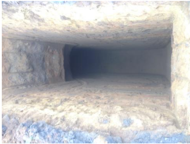
Photo 49: Excavation of trial pit TP09.
