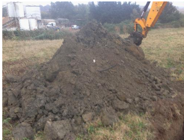
Photo 64: Arisings from trial pit TP16.
