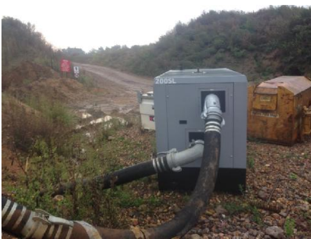
Photo 7: View of access route into eastern area of Area 1, with water pump in the foreground.
