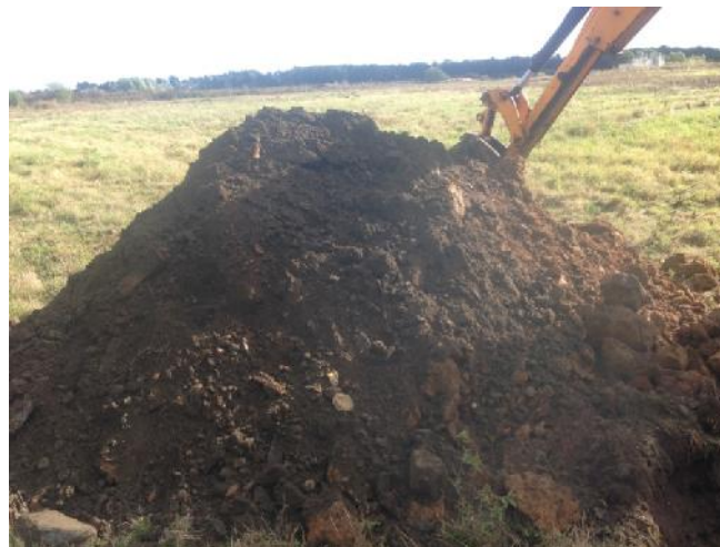
Photo 80: Arisings from trial pit TP25.
