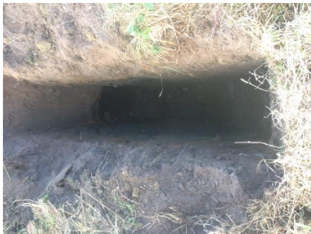
Photo 77: Excavation of trial pit TP24.
