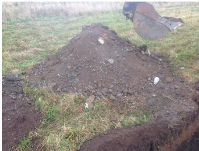
Photo 74: Arisings from trial pit TP22.
