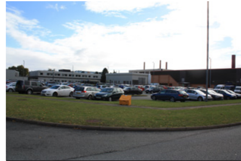
Office complex and parking
