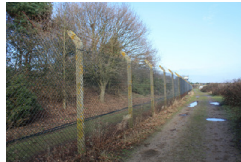
High security fencing
