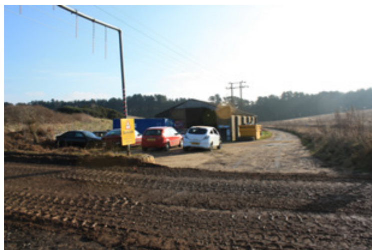
Concrete unit to the centre west of the area
