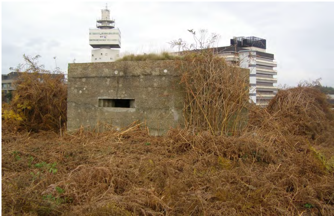
Figures 7.3 and 7.4 The Scheduled barrow surmounted by a pill box
