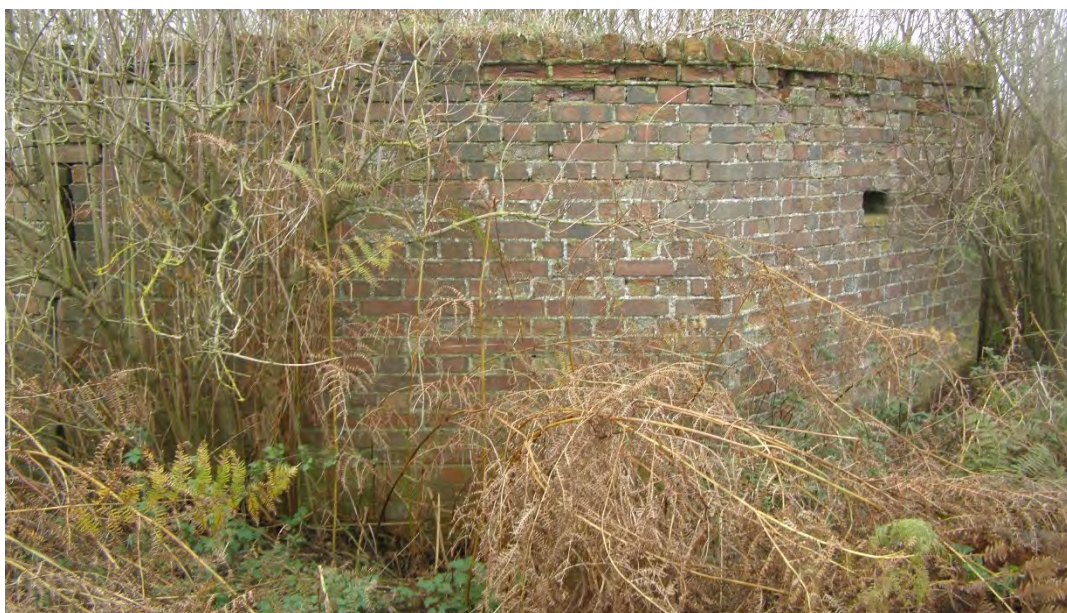
Figure 7.15 The octagonal brick base today
