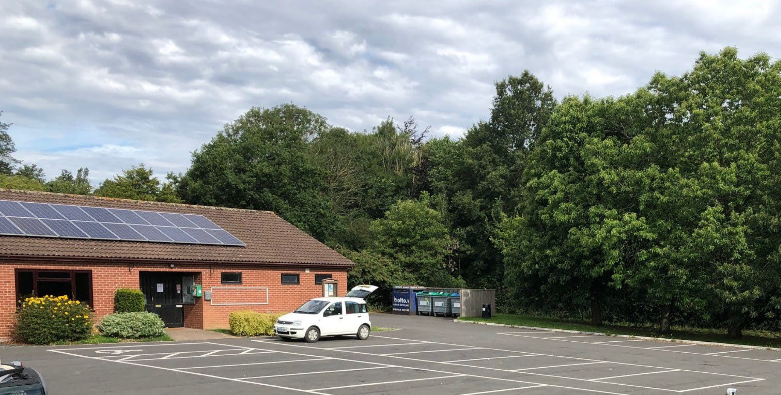
Ufford Recreation Ground Car Park Resurface
