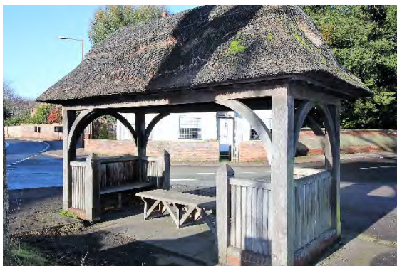
Jubilee Shelter, Brook Street of 1935.
