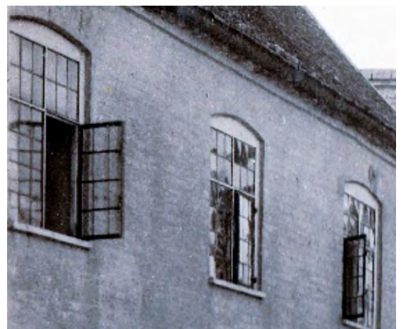
Typical Casement Windows at Haven House, now removed
