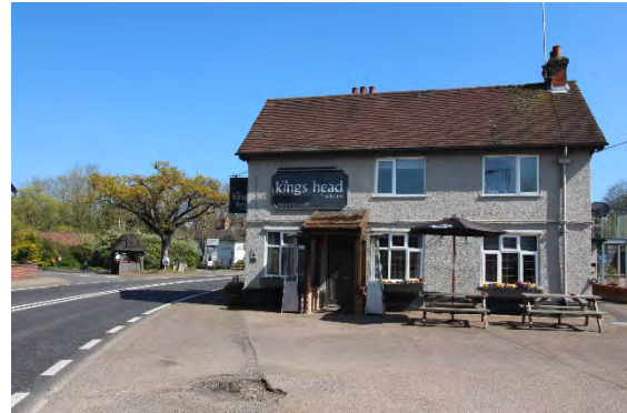
The southern elevation of the King's Head showing replacement windows
