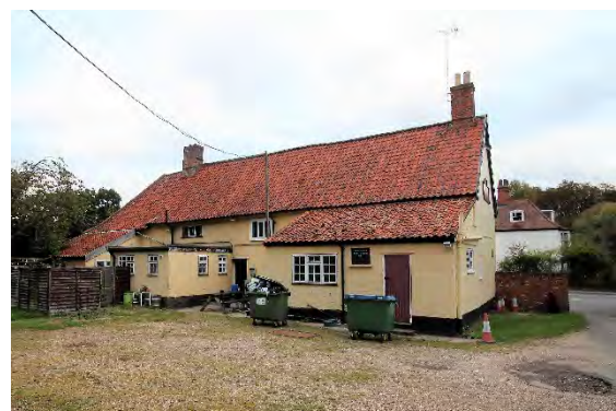
Car Park Elevation of the Griffin Inn, High St
