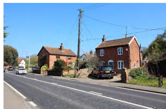
Bourne Cottage and Brewers Cottages, Brook Street, survivors from a cluster of labourers' cottages built just to the south of The Kings Head c1820. Brewers Cottage has been partially rebuilt.
