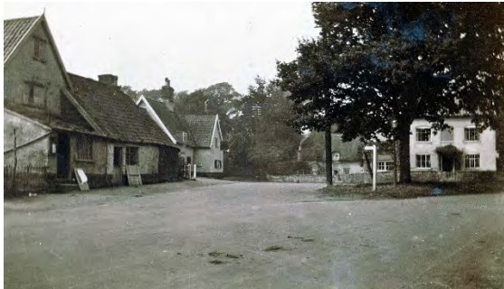
The now demolished wheelwrights and stables at the Kings Head c1920
