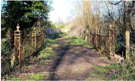
Bridge over former drive to Cockfield Hall, High Street
