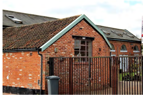
The Western elevation of No.26 High Street
