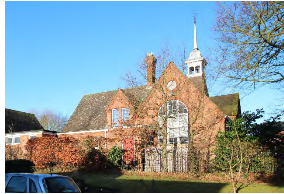
Oakwood Park façade of Yoxford School
