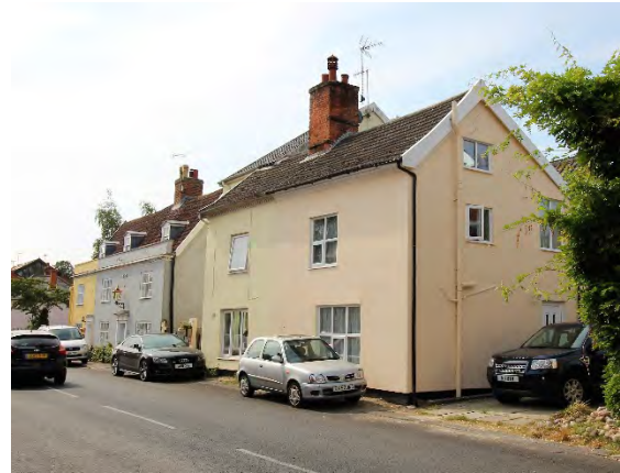
Yew Tree Cottage and Yew Tree House, High Street
