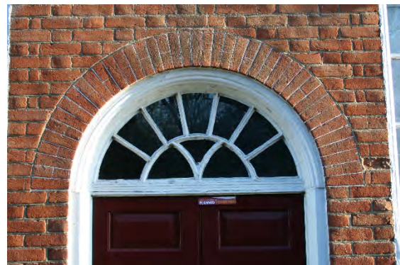
Detail of fanlight, Chapel House
