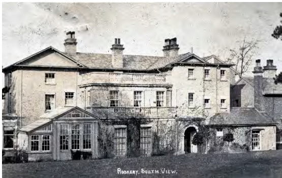
Southern façade of The Rookery
