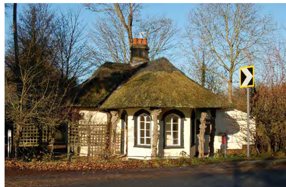
The GII listed Darsham Road Lodge to Cockfield Hall
