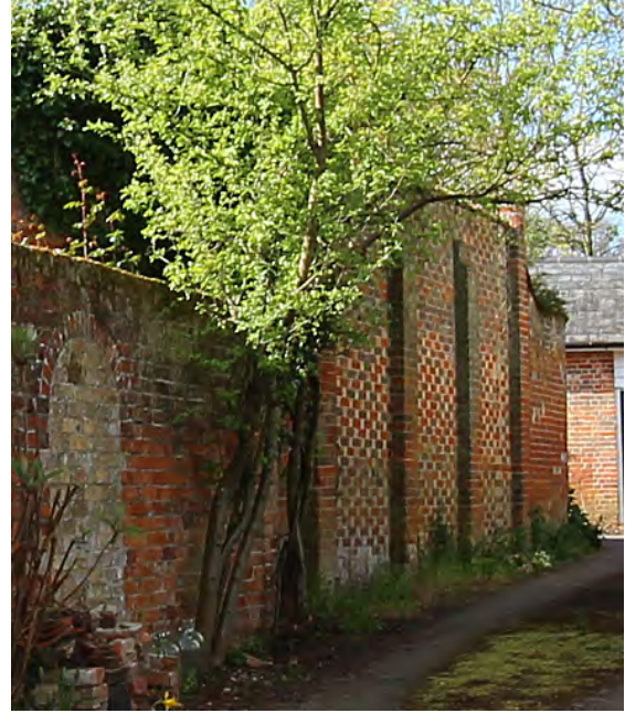
Magnolia House garden walls to the rear of Haven House
