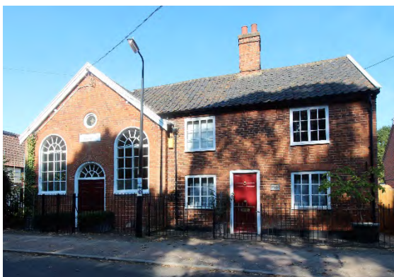
Chapel House, High Street
