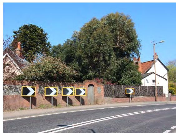
Signage and street lighting west side of Brook Street
