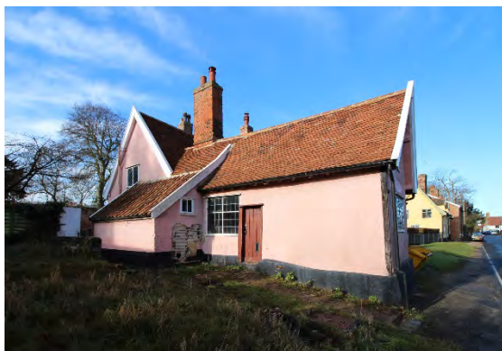
Wisbech Cottage, High Street
