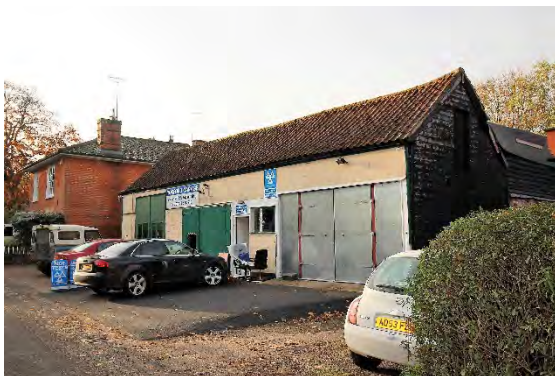
Yoxford Garage, Old High Road
