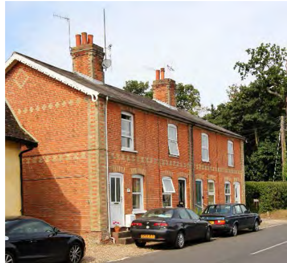
Nos. 1-4 (cons) Hope Cottages, High Street
