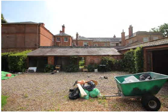
Service courtyard to rear of Grove Park
