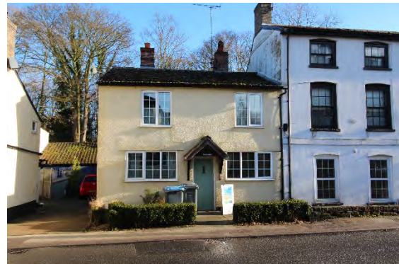
Taywood Cottage, High Street
