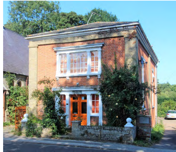
Former Methodist Chapel, High Street c1833-35
