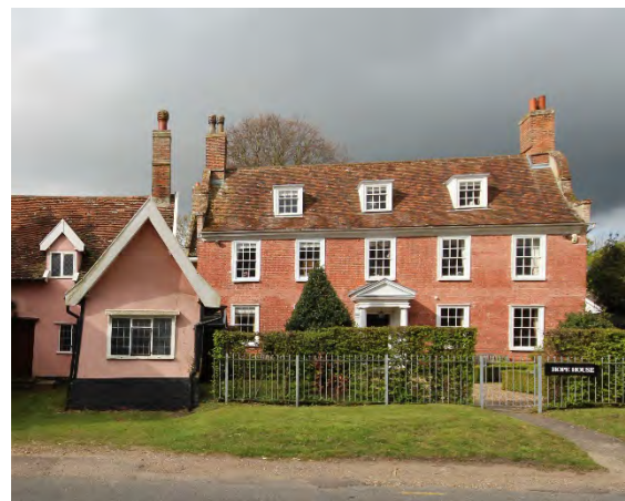
Early eighteenth century brick façade, Hope House
