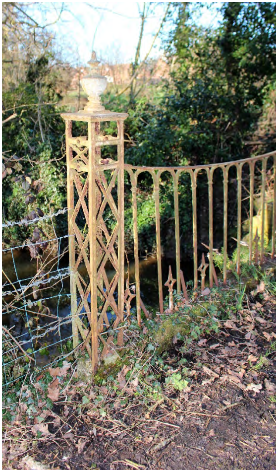
Detail of pier, Bridge over former drive to Cockfield Hall, High Street
