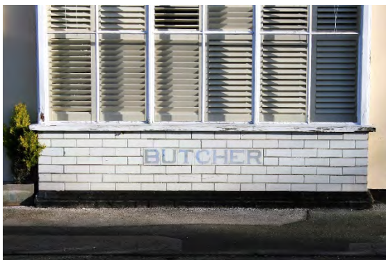
Early twentieth century shop front Garden House
