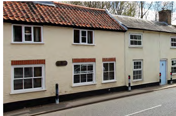
Bollards on the north side of High Street.
