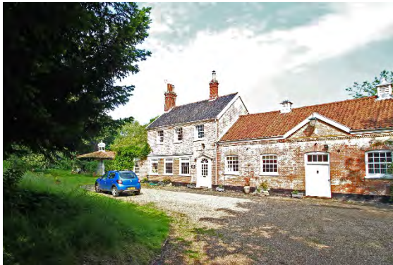
Former Stable, Coach House and Kennels, Grove Park
