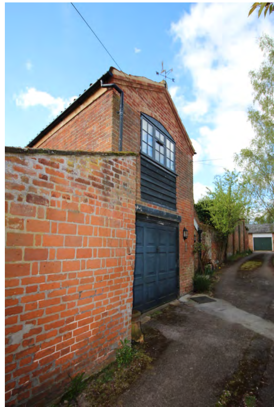
Converted Workshop to rear of Milestone House
