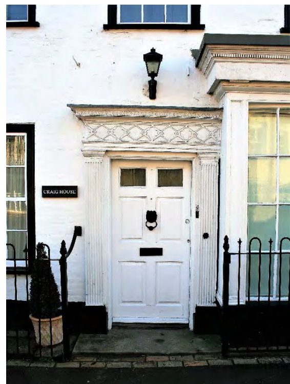
Fine mid eighteenth Century doorcase and early nineteenth century shop fascia at Craig House, High Street
