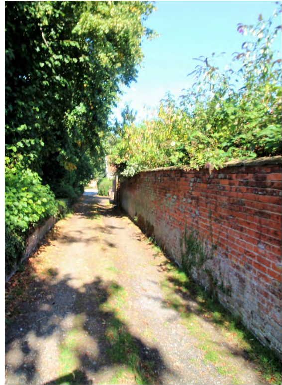
Garden wall to ‘Cleghorns’ on Church Lane looking north.
