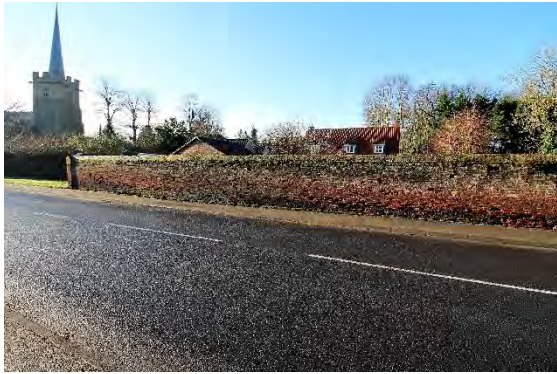
Wall to Bowling Green of the Former Three Tuns Hotel, High Street
