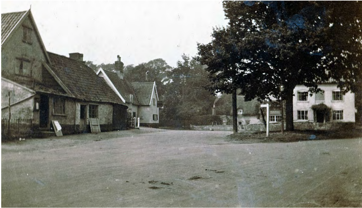
The now demolished wheelwrights and stables at the Kings Head c1920, in the centre ground are the Thatched Cottage and Dickory Cottage now hidden behind a high later twentieth century wall, on the right Bank House.
