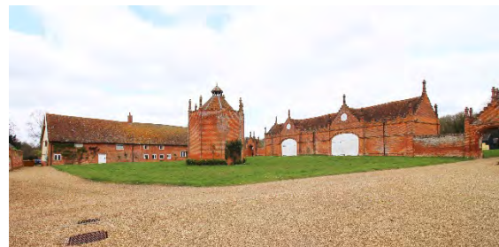
Three Grade II listed stable court buildings at Cockfield Hall
