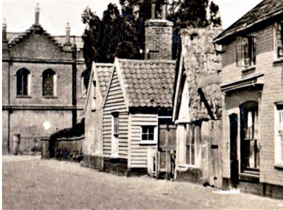
Pan tiles thatch and weatherboarding on demolished cottages, High Street c.1920
