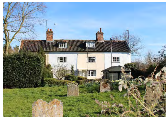
Nos.1-4 (cons) Church Lane, from the churchyard
