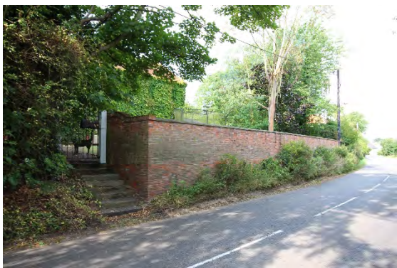
Little Street Boundary Wall to Yoxford Place
