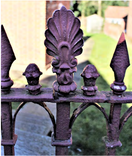
Detail of nineteenth century railings, Cockfield Hall Lodge, High Street
