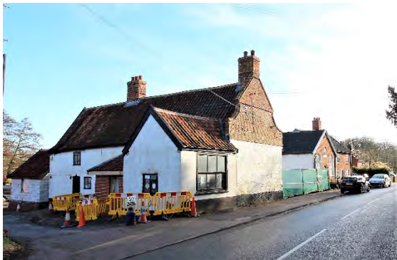
Nineteenth century former shop to the rear of the Coal Yard House
