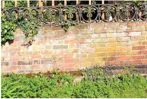
Wall and Railing to rear of the Old Schoolroom
