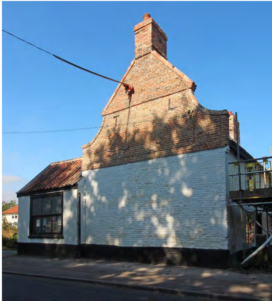
Later seventeenth century brickwork, Coal Yard House
