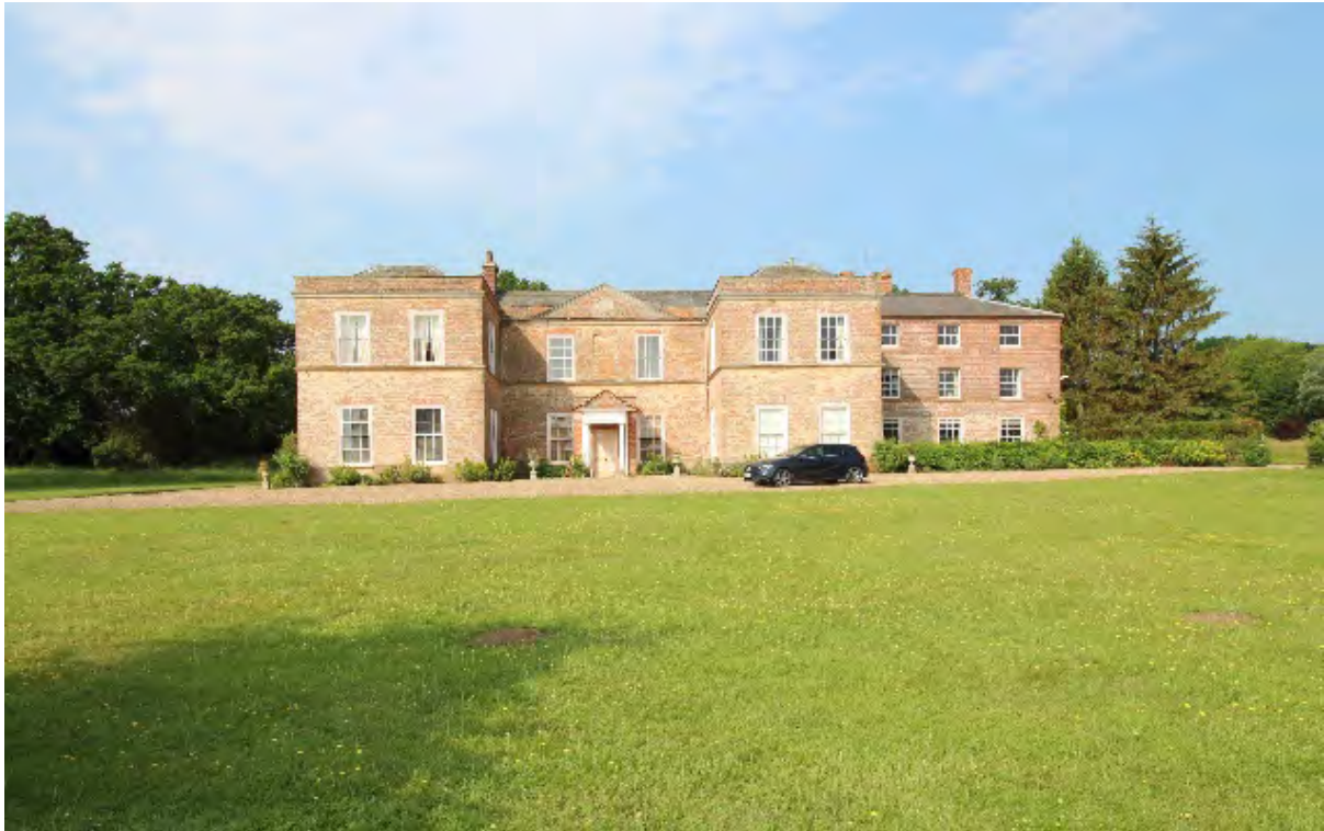
Grove Park, south elevation
