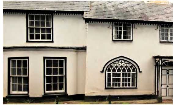
Early nineteenth century and later replacement windows, The White House, Brook Street
