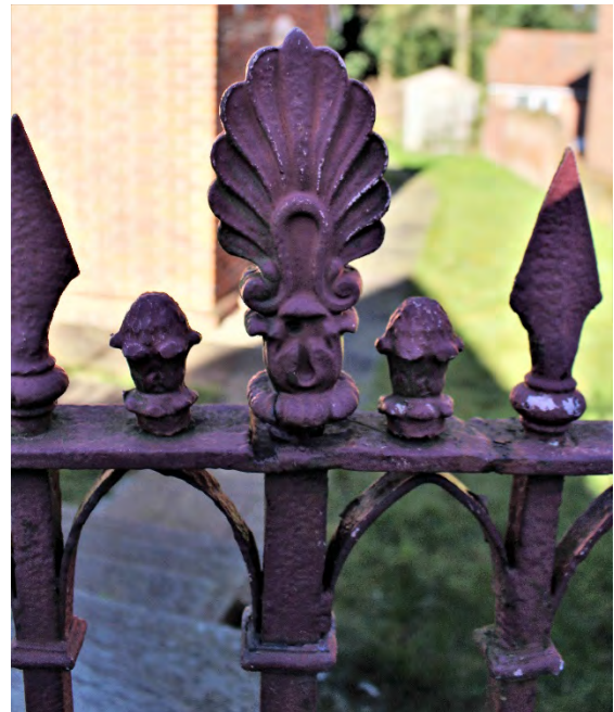
Detail of railings to Cockfield Hall's lodges
