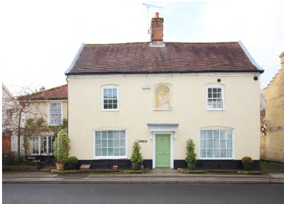
Haven House, High Street
