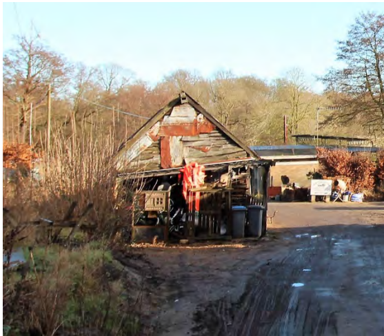
Outbuilding at Coal Yard House
