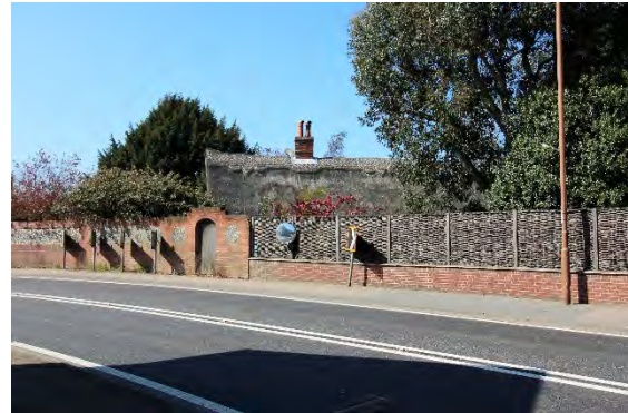
Thatched roof of Thatched Cottage and Dickory Cottage rising above the high boundary wall and fence to Brook Street
