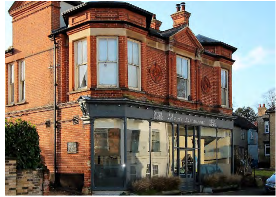
Blythburgh House's shopfront of c1902 has been adapted but remains largely intact.
