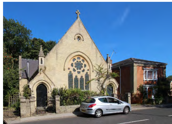
Chapel House, High Street
