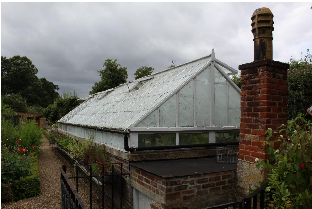
Figure 17 Greenhouse with boiler
