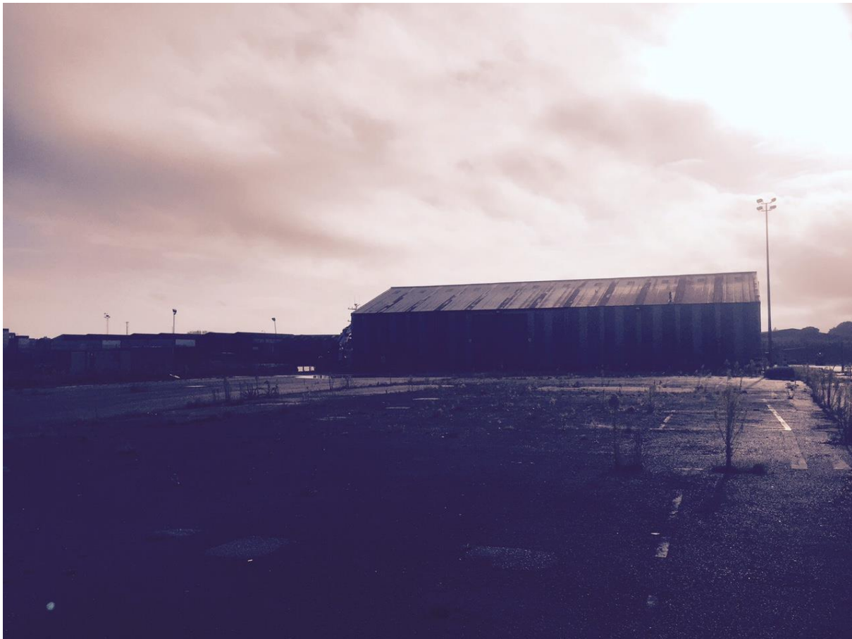
Figure 33 – Land adjacent to former Shell Building – view across site towards slipway
