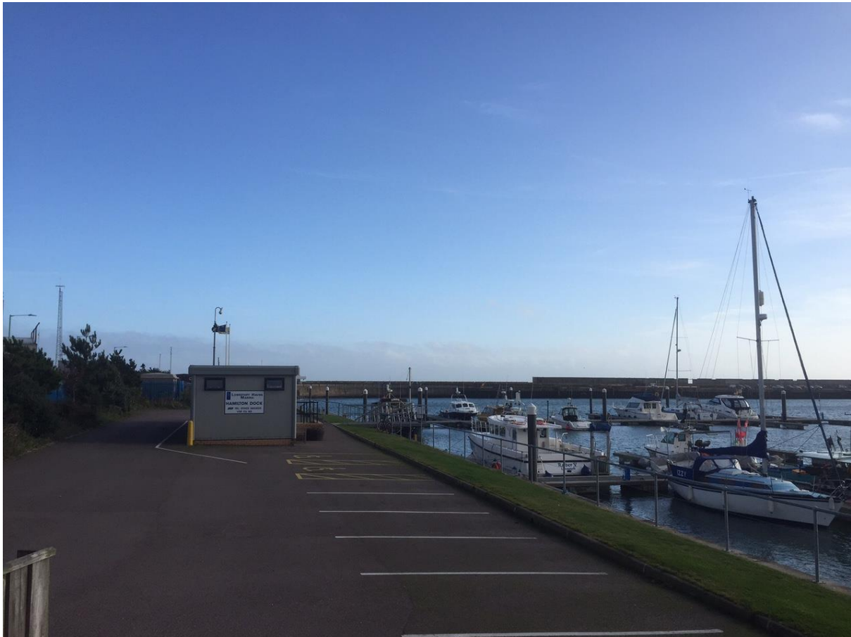
Figure 18 - Site 1 - Hamilton Dock North
