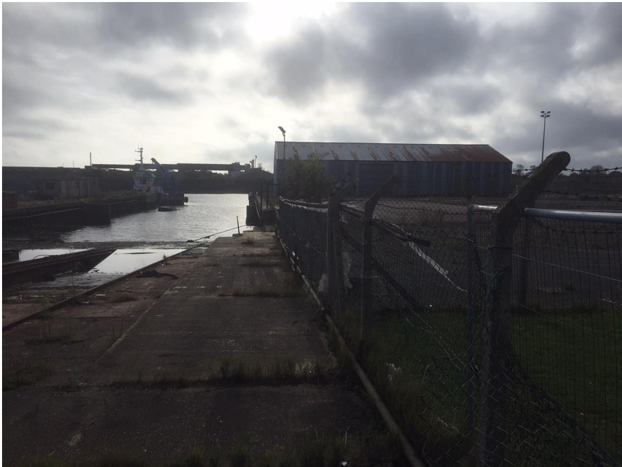
Figure 34 - Land adjacent to former shell building showing existing slipway
