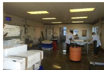
Figure 12 - Processing area within Fish Merchants premises (note suspended ceiling)
