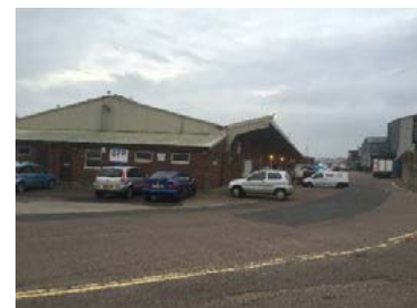
Figure 9 - Auction offices and toilets at end of Fish Market building
