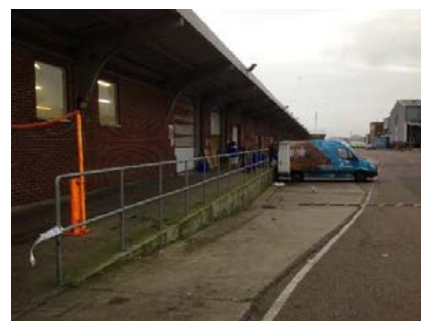
Figure 8 - Roadside loading bay facilities along western elevation of Fish Market
