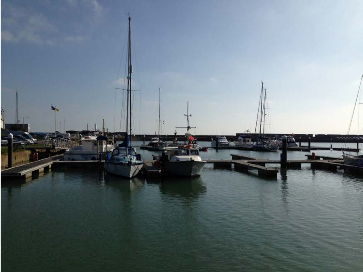
Figure 16 - Looking towards Site A showing existing pontoons in Hamilton Dock
