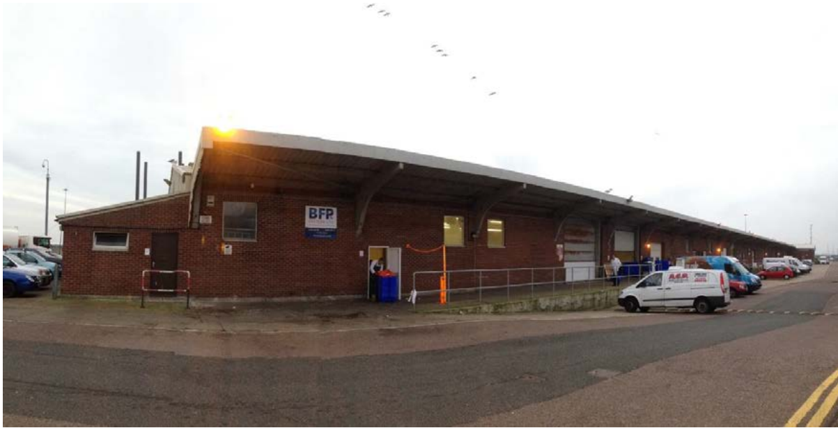
Figure 26 - Existing fish market
