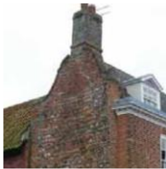
Coursed brick and flint in a gable, Northgate
