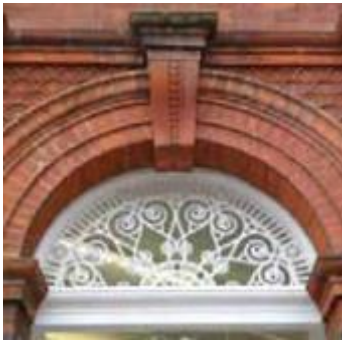
Moulded brickwork and cast iron, Smallgate
