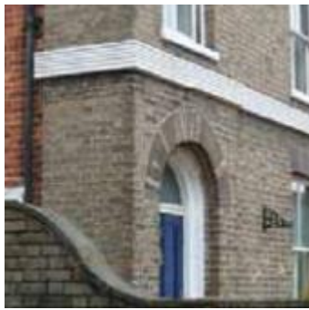
Gauged brick arches and a reeded string course, Station Road
