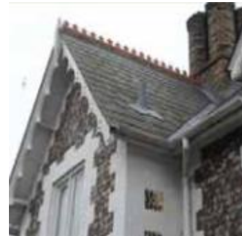
Painted brick and course, knapped flintwork with decorative bargeboards, slates and chimney stack, Puddingmoor
