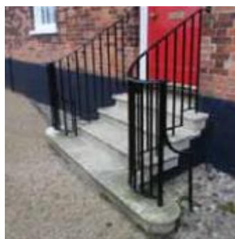
Stone steps and metal handrails, Northgate
