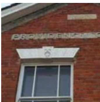
Stone details and cast iron flat arches, London Road
