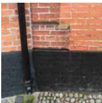
Brickwork quoins, cast iron downpipes and flint cobble surfacing, Northgate
