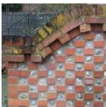
Red brick and flint cobble combined in a modern wall, Puddingmoor
