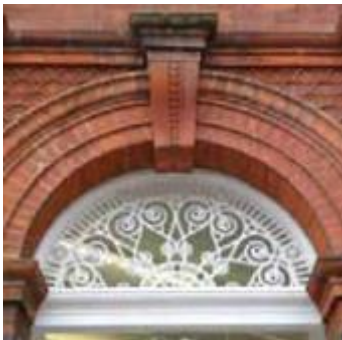
Moulded brickwork and cast iron, Smallgate
