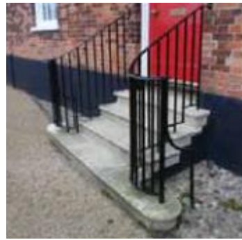
Stone steps and metal handrails, Northgate
