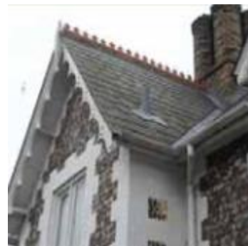
Painted brick and course, knapped flintwork with decorative bargeboards, slates and chimney stack, Puddingmoor
