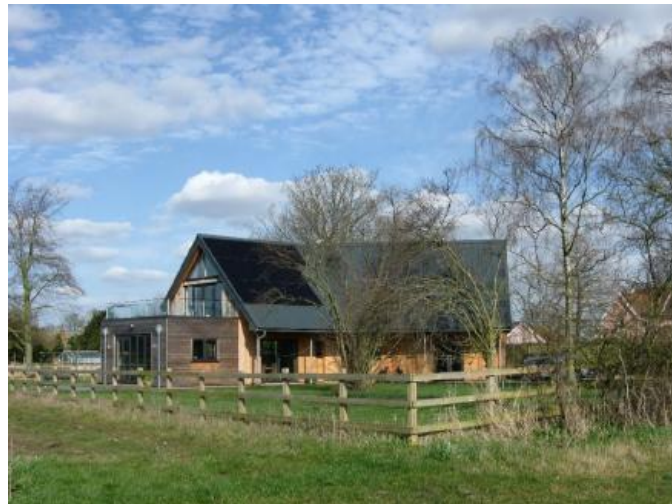
New build Belvedere.
