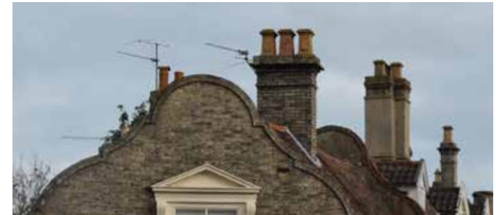
Roof and chimney detail
