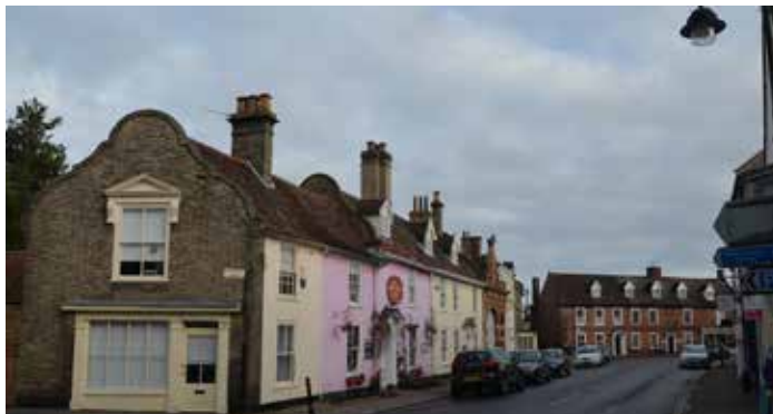
Two storey dwellings in Earsham Street
