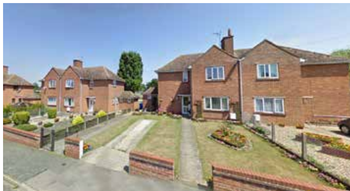
Semi - detached houses on St John's Road
