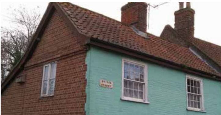
Variety of materials and colors on the facades
