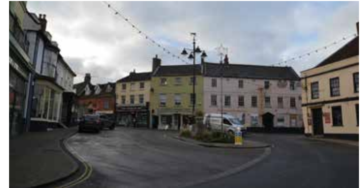
Three storey dwellings in Earsham Street
