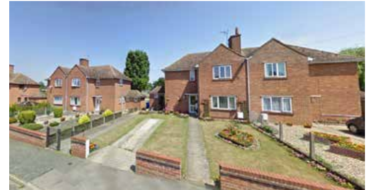
Two storey dwellings in St John's Road
