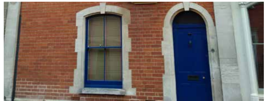
Painted doors and windows
