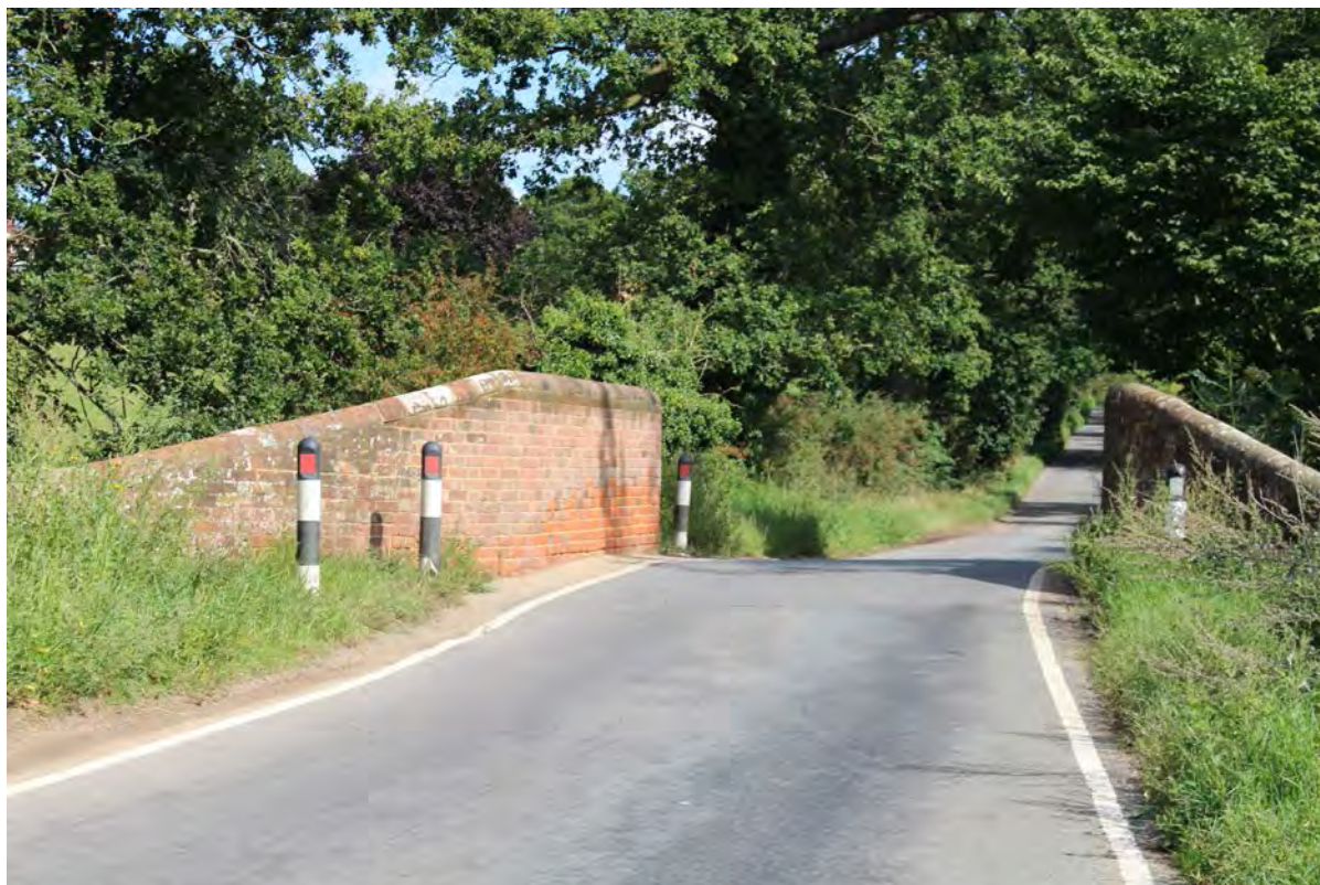
Boot Street bridge
