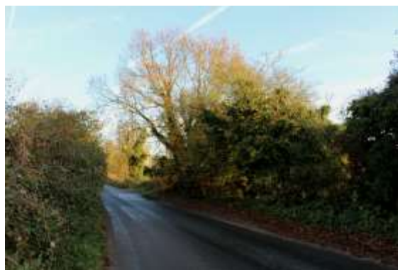
Towards Boot Street Bridge from the west
