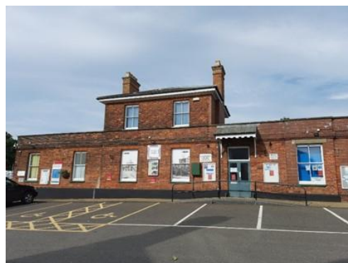
Halesworth Railway Station
