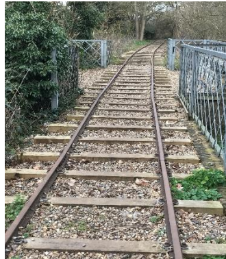
Relaid track over the bridge
