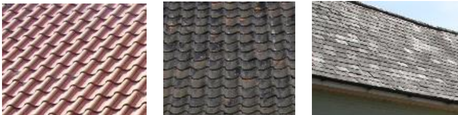
Different types of roof tile in Halesworth
