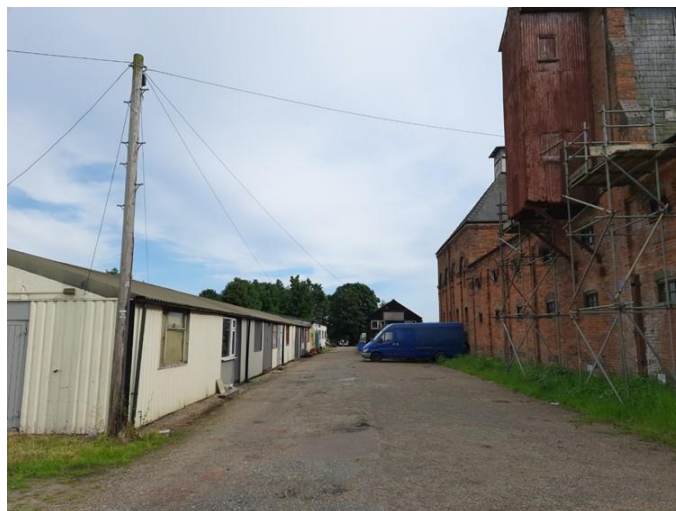
Workshops at Station yard with a Maltings building opposite
