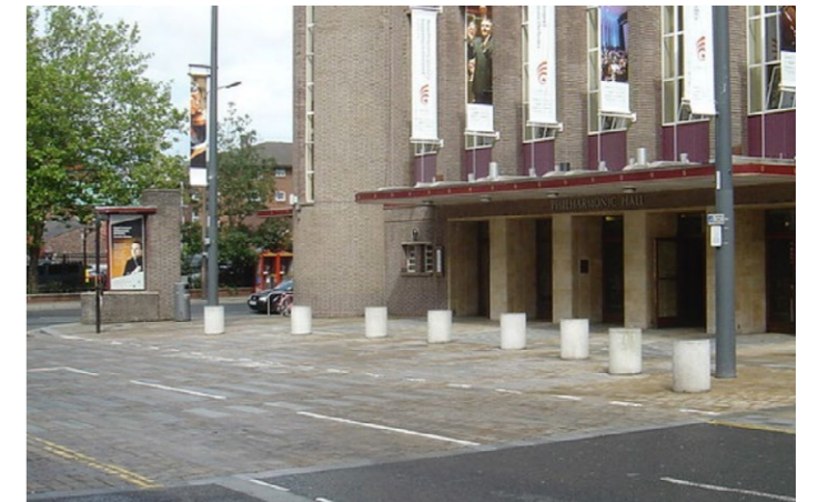
Footway treatments extended across the carriageway to highlight an entrance
