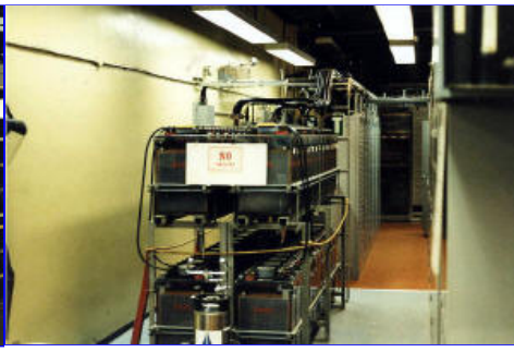
Battery Backup System on the right, the cabinets housed the AC to DC rectifiers, DC to AC converters, along with voltage regulators.
