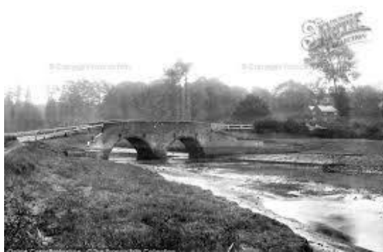
Wilford Bridge, 19 th century
