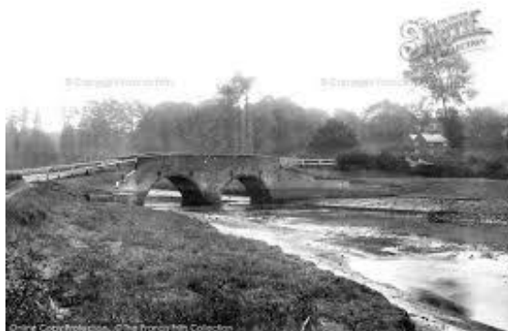
Wilford Bridge, 19 th century
