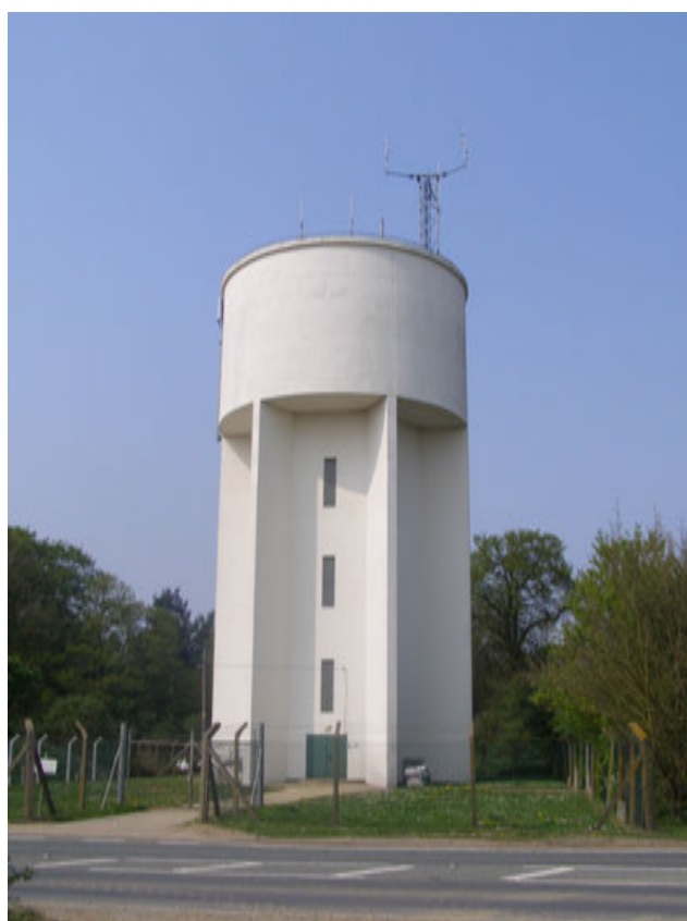
The water tower, A1152
