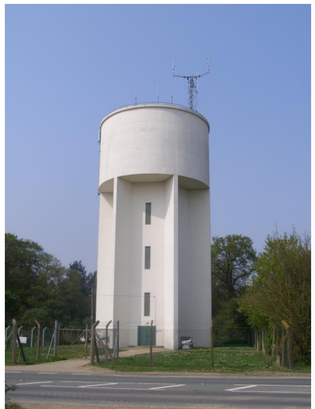
The water tower, A1152
