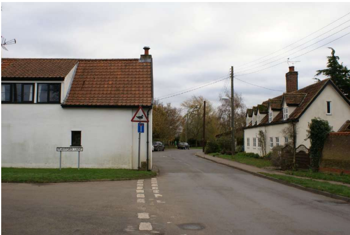
View along illustrating historic cottages at Junction with Playford Lane
