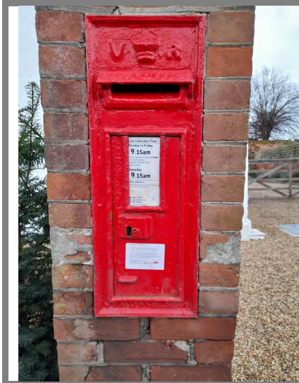
Figure 46: Victorian Post-box at South entrance
