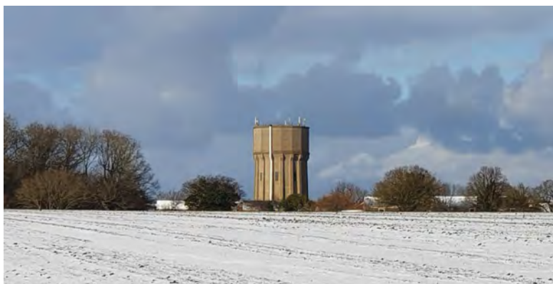
Figure 42: The Water Tower, Rendham Road.
