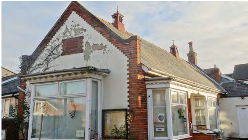
Figure 41: The Gannon Institute, but generally known as The Gannon Rooms.
