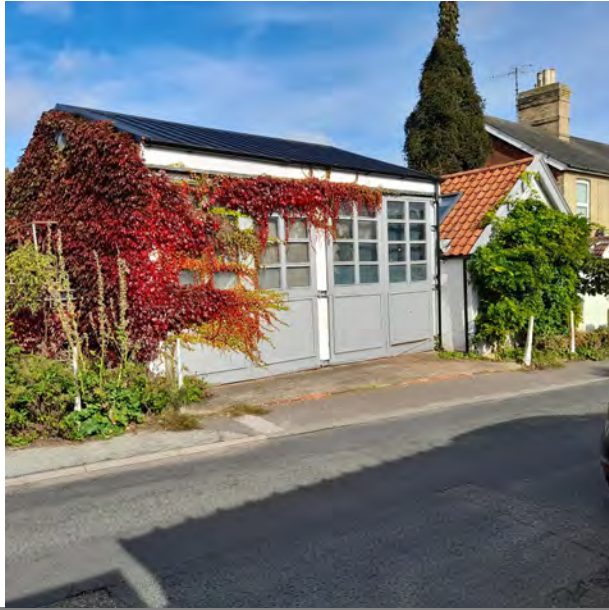
Figure 34: The Old Fire Station, Rendham Road.
