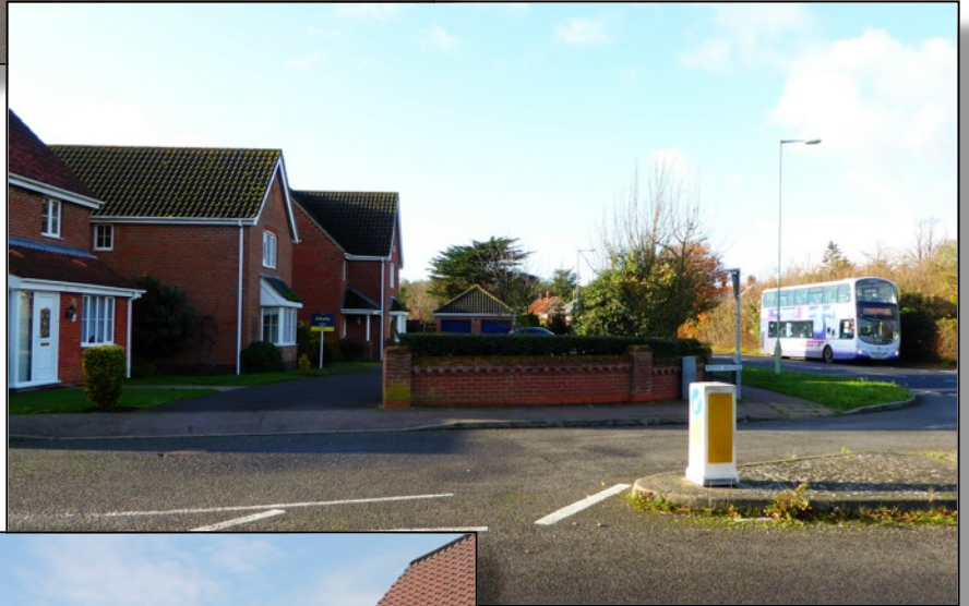
Access to the development from the Lowestoft Road.
