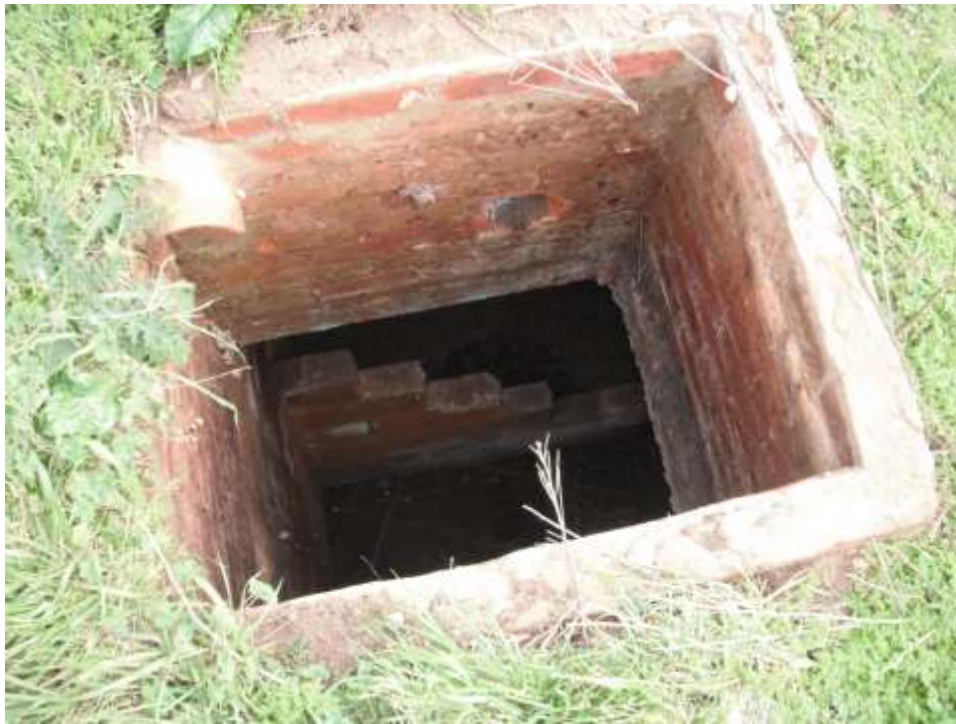
Figure 9: Open manhole leading to an underground tank.
