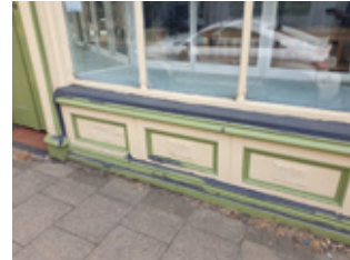
Example of paneled stallriser on traditional shopfront.
