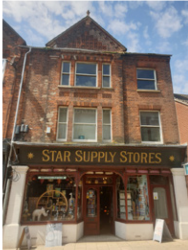
Example of shopfront with 'A' framed board outside the entrance, along the pedestrian walkway.
