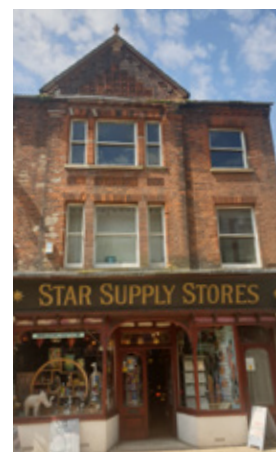
A traditional shop-front making use of the glazed front windows to display its good and products. Again the shop-front is appropriate for the building.
