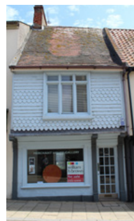
A shop-front and building working as one single element. The colour scheme, detailing and design are appropriate for this building.
