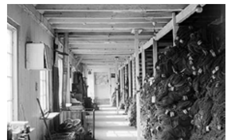
Interior of the Netting Sheds ©English Heritage NMR Reference Number: AA98/12838
