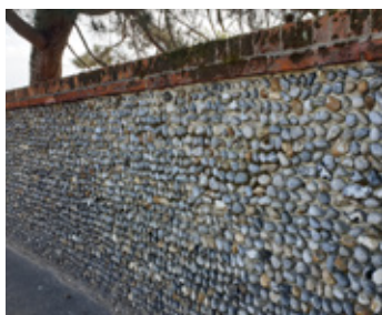
Pebble wall with red brick coping
