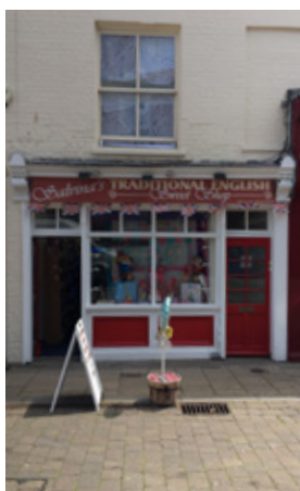
Another traditional shop-front with a co-ordinated colour scheme, signage and window display. See this guidance for further advice notes on the appropriate use of A boards.
