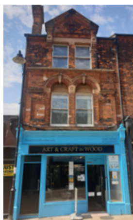
This traditional shop-front is an example of a business applying its branding to a restored structure. Colour choice should be approved by the Local Planning Authority.
