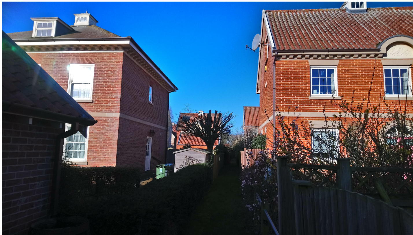
Existing similar houses on adjacent development at Garden Square
