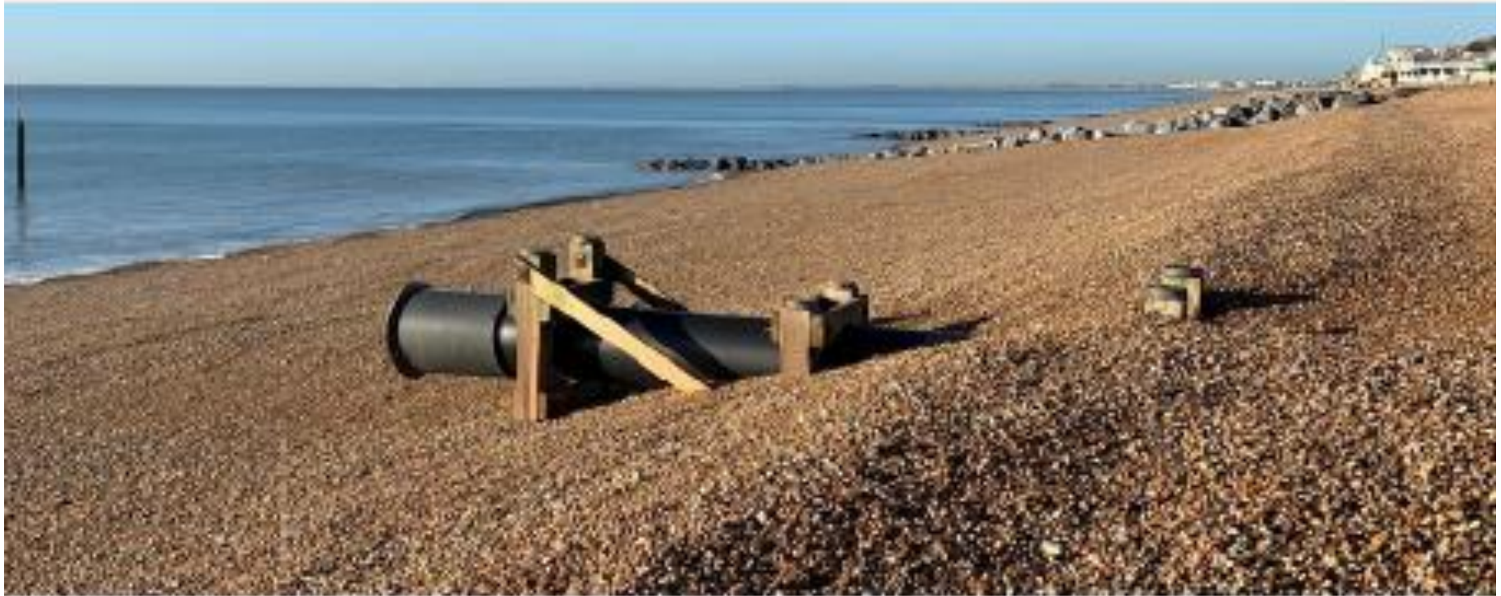
4.17 Example image of a similar marine outfall
