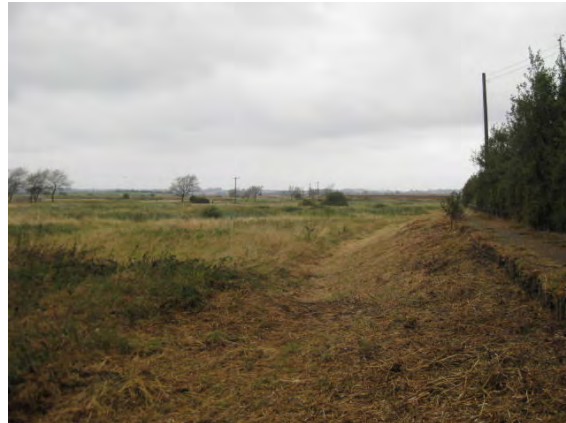
Strimmed bank: reptile mitigation prior to EA bank strengthening works by EA
