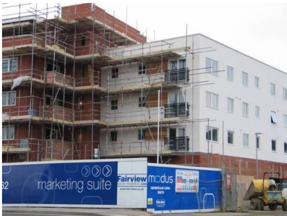
Waterside (Ipswich) apartments nearing completion.
