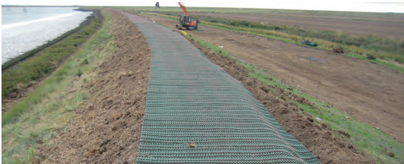
Trial upgrading work on the Orford wall, west of the Quay before grass seeding.
