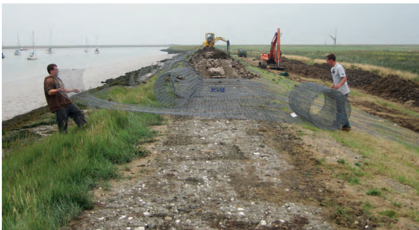
Trial upgrading work on the Orford wall, west of the Quay.
