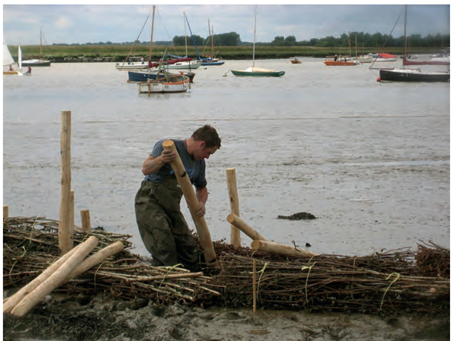
Installing faggots for the saltings regeneration project at Iona site Aldeburgh.
