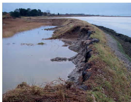
Damage and breaches to Hazlewood Marsh wall after the surge tide December 2013.
