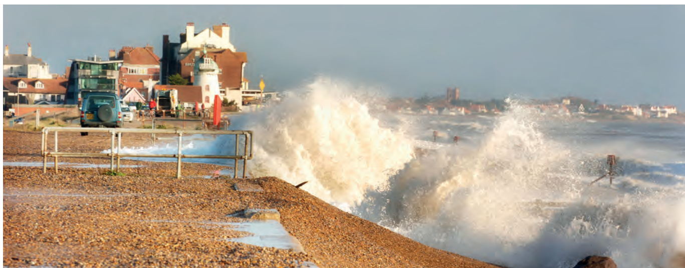
20 Sea wall at Slaughden under pressure at high tide.
