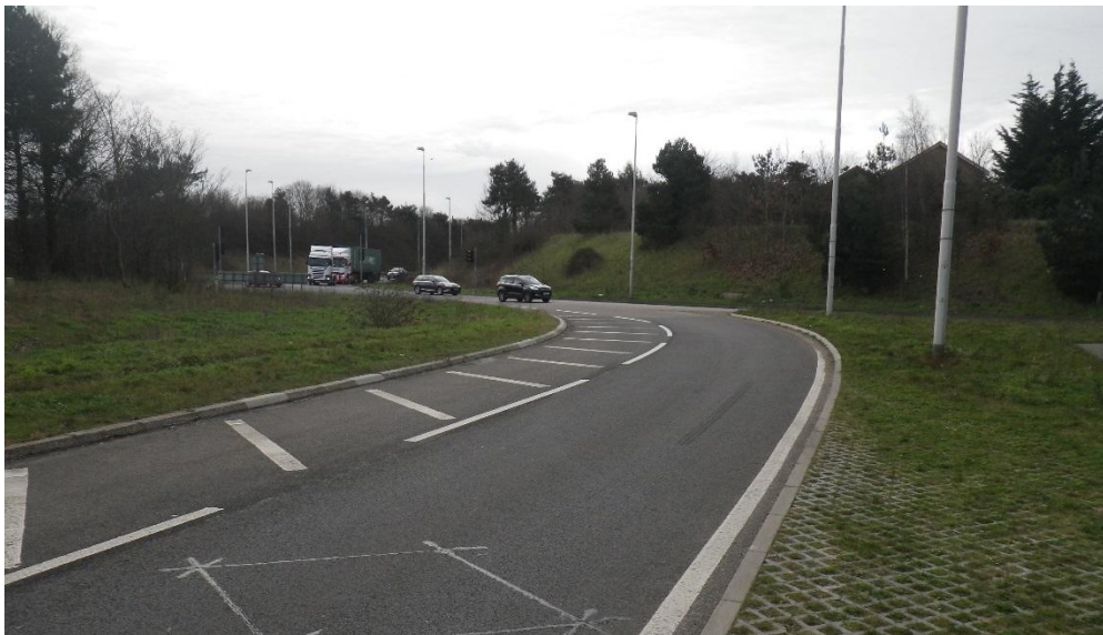
Photograph 5: Westside circulatory carriageway
