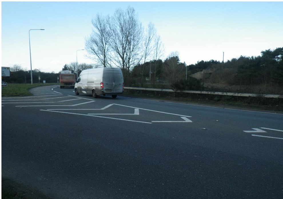
Photograph 4: Junction 58, south side circulatory carriageway
