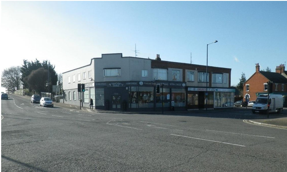
Photograph 10: Junction viewed from the Garrison Lane/High Road West southwestern corner
