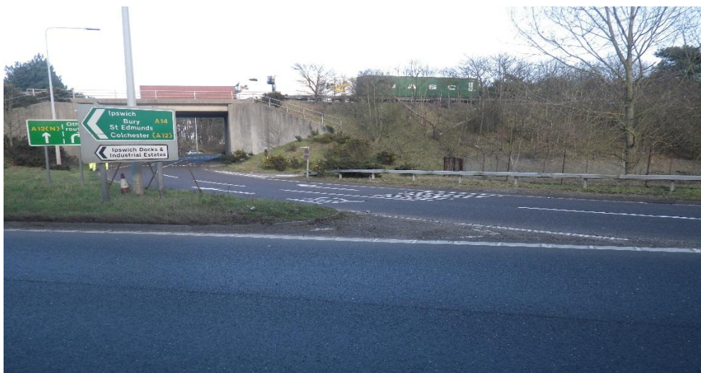
Photograph 1: Junction 58 viewed from the start of the A14 westbound on-slip
