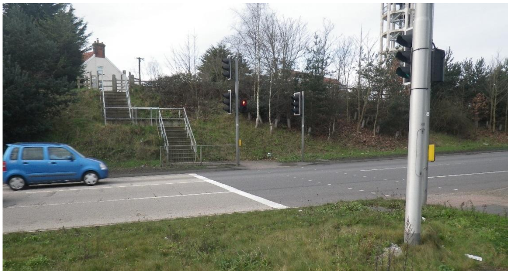
Photograph 7: A14 exit slip road with pedestrian crossing leading to the Trimley St. Mary residential area
