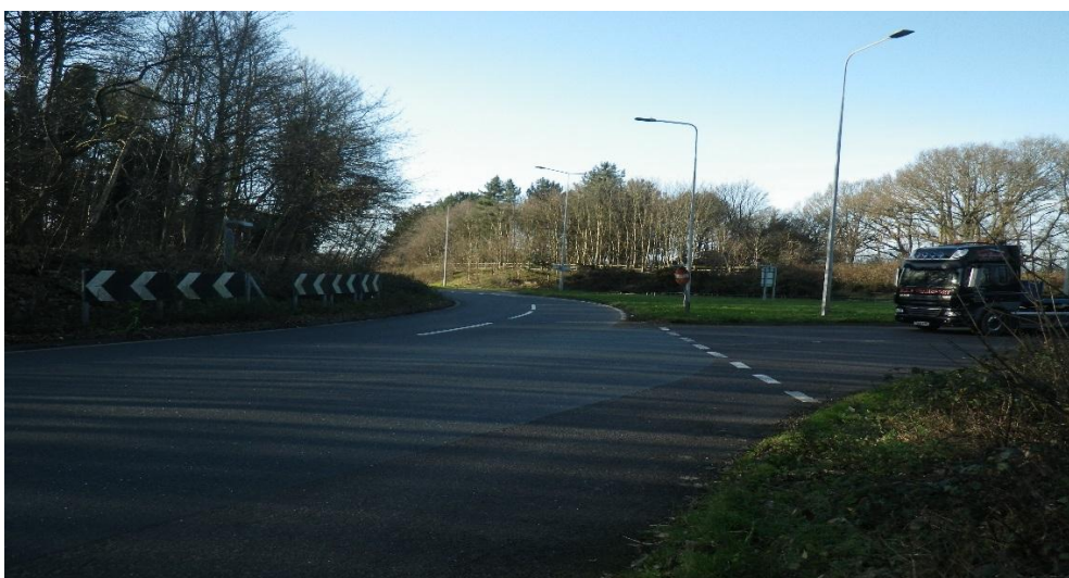
Photograph 2: Junction 58 viewed from the intersection of the roundabout and the A12 southbound
