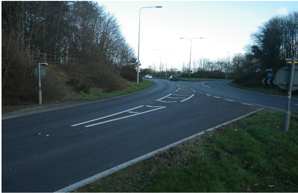
Photograph 3: Junction 58, A14 eastbound off-slip
