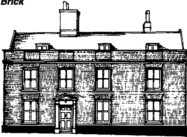
A number of timber framed buildings were refaced in brickwork during the 18 th century.
