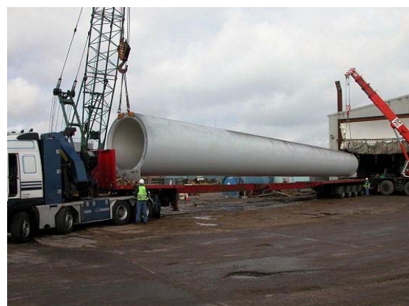
Figure 5-4: Moving Upper Tower Section
