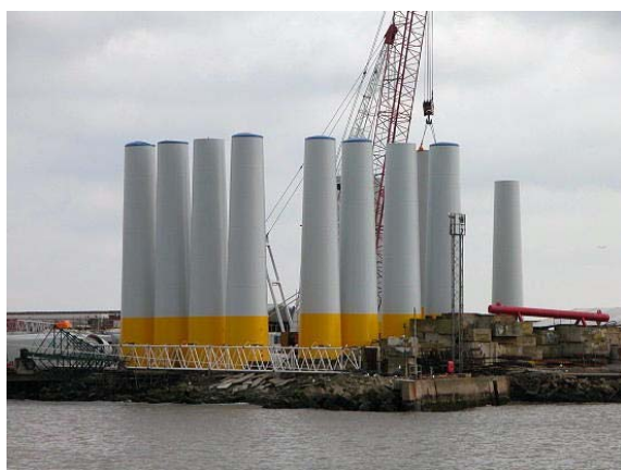
Figure 5-3: Tower Storage at Lowestoft
