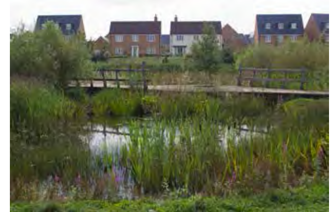
Drainage pond forming part of a wider SUDs network
