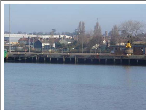
Photo 0-7 Revetments with a hollow quay deck north bank
