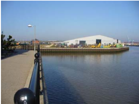
Photo 0-23 Sheet piling along Kirkley Water Front
