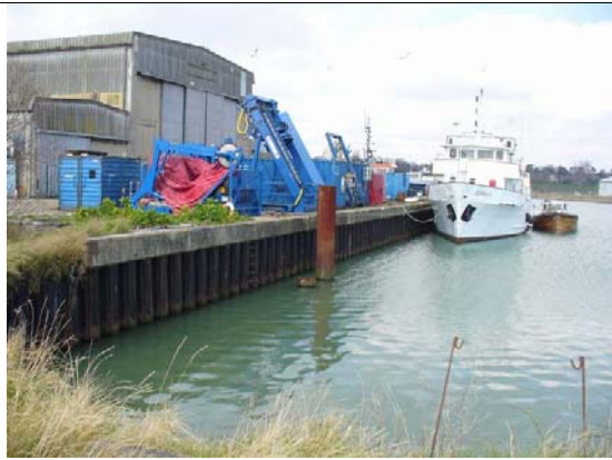
Photo 0-28 Sheet piling with concrete capping in front of Brooke Marina looking west
