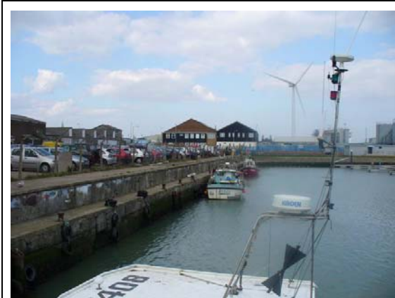
Photo 0-11 Concrete wall inside Hamilton Dock
