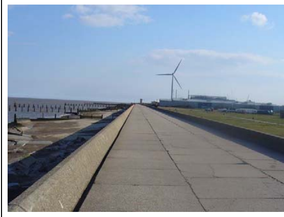
Photo 0-15 Seawall further north with groynes looking south
