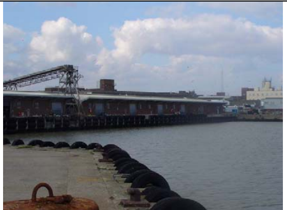
Photo 0-10 Steel sheet piling with concrete capping
