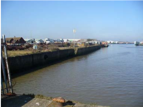
Photo 0-19 Concrete on south bank near Bascule bridge looking west along South Quay
