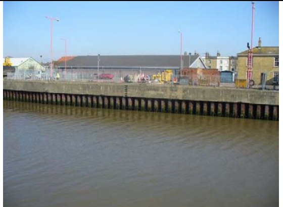
Photo 0-8 Steel sheet piling with concrete capping, north bank
