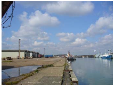
Photo 0-24 Raised quay crest with sloping ground
