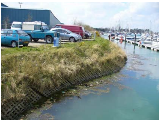
Photo 0-29 Revetments along School Road Quay looking west
