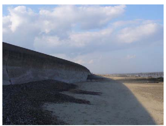
Photo 0-16 Unprotected seawall toe looking north
