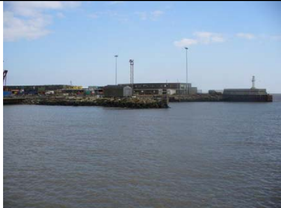
Photo 0-12 Undefended areas inside Waveney Dock along the North Pier Extension
