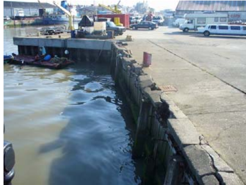
Photo 0-20 Deterioration of defence wall along South Wharf looking east
