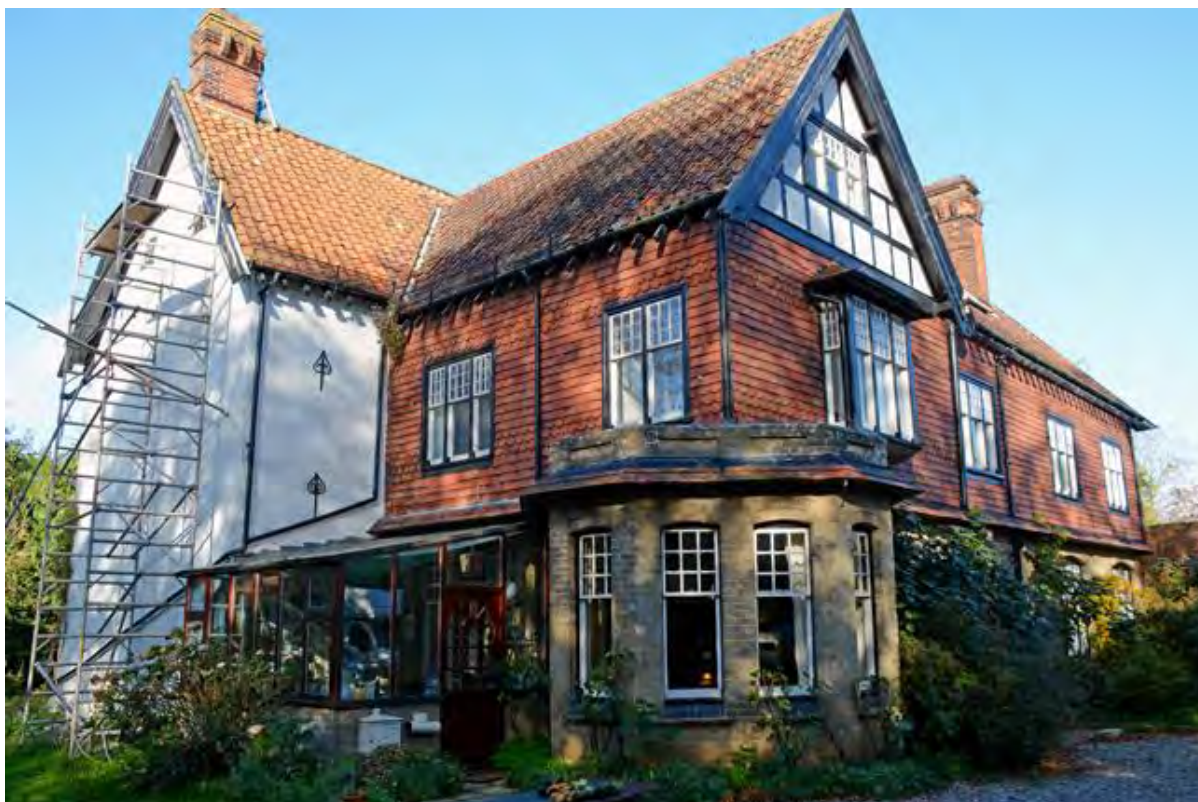
Manor House : Late C19 extension looking to north west
