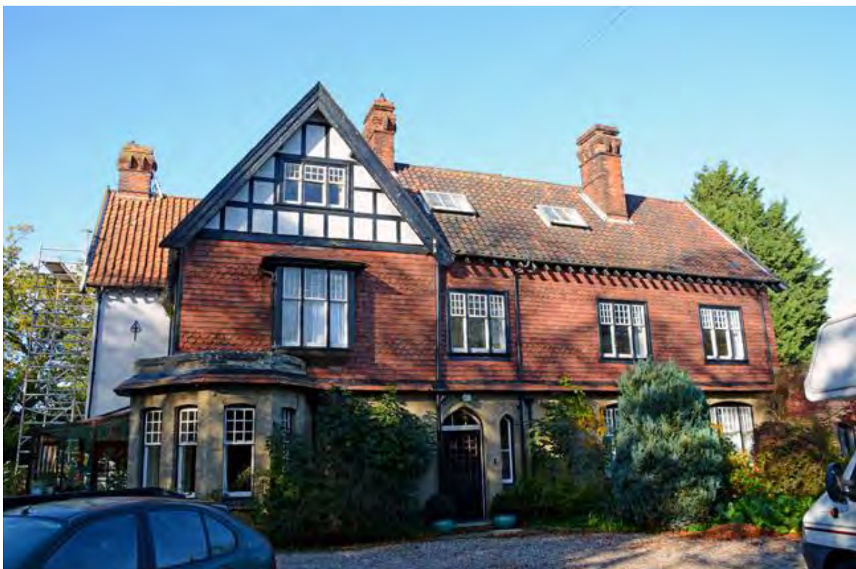
Manor House : East elevation of the late C19 extension
