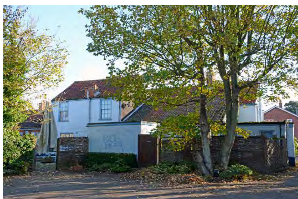
27 : Rear of the building looking east
