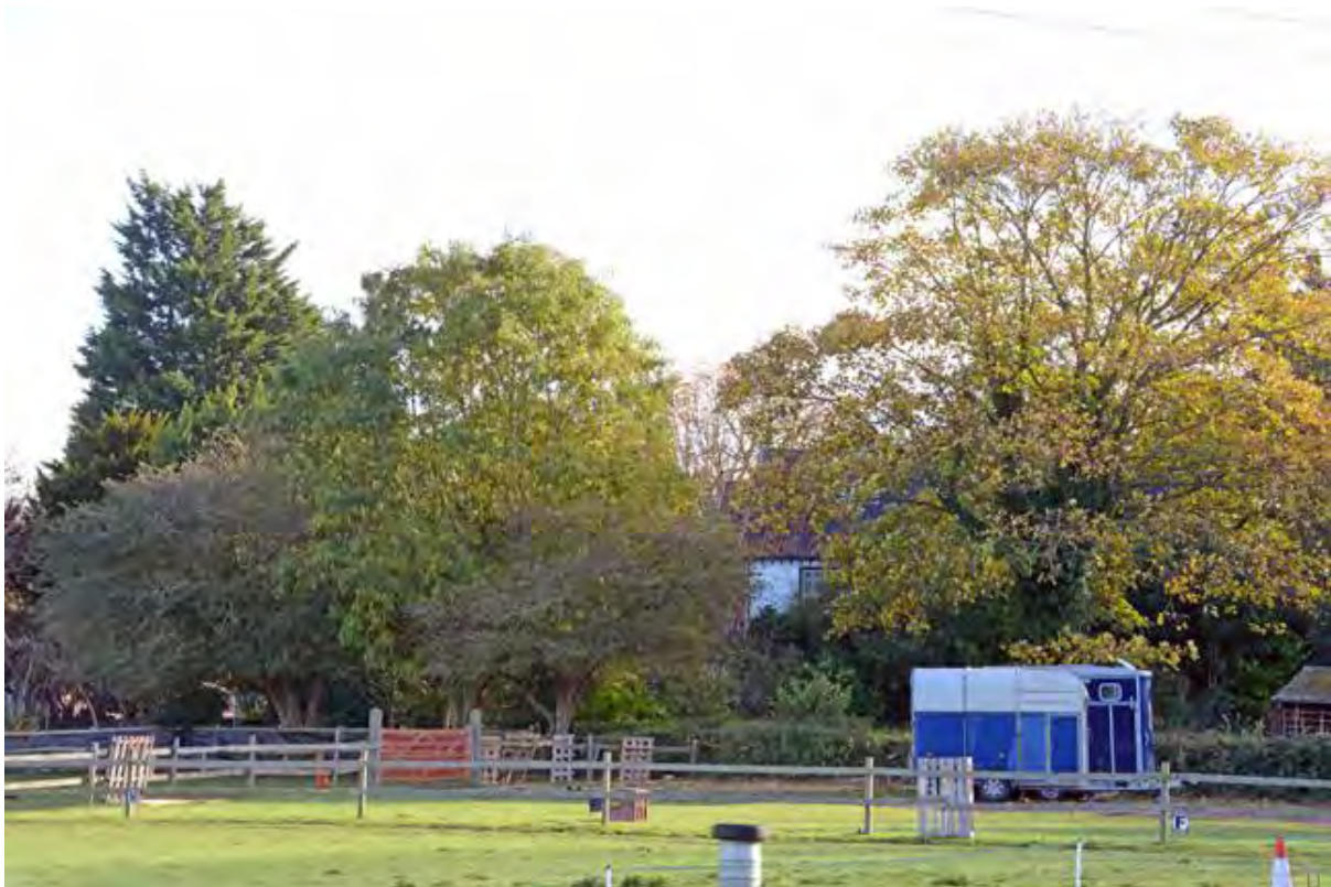
20 : Closer view looking to east, also in October, where the building is seen through the trees. During the winter months a greater extent of the building becomes visible.
