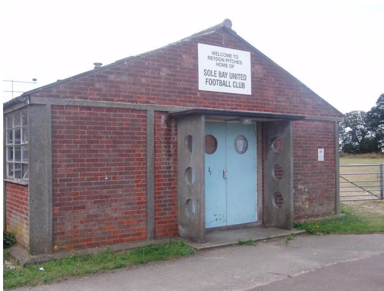
Poor quality changing facilities at the former Reydon High School Site
