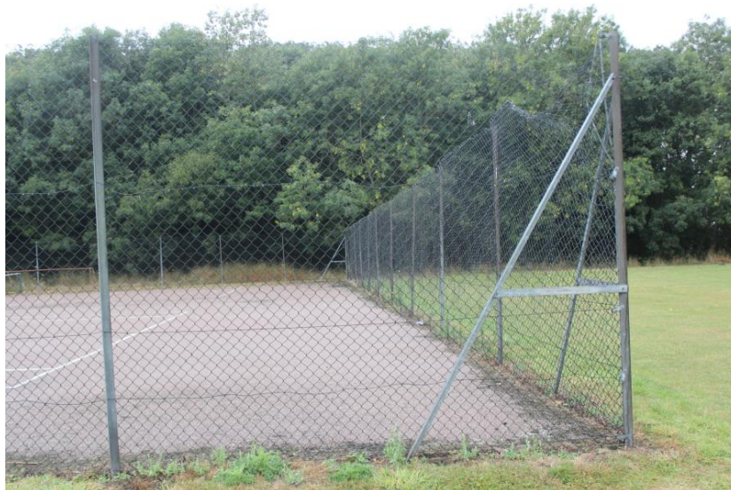
Poor quality tennis courts at Ringsfield
