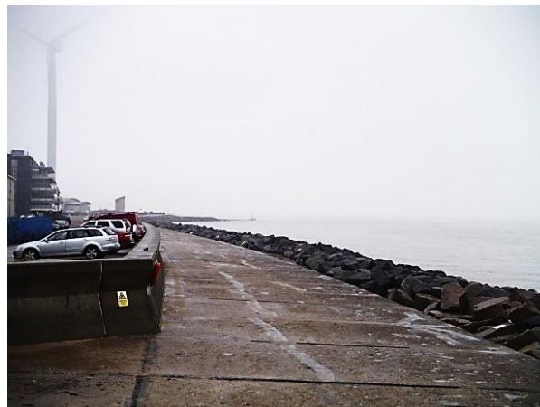
Figure 1-2 - Example of sea wall along the PowerPark site (source: AECOM, December 2017)
