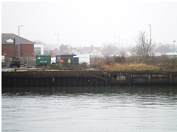
Figure 1-1 - Example of river wall along the Kirkley Waterfront and Sustainable Urban Neighbourhood Site (source: AECOM, December 2017)
