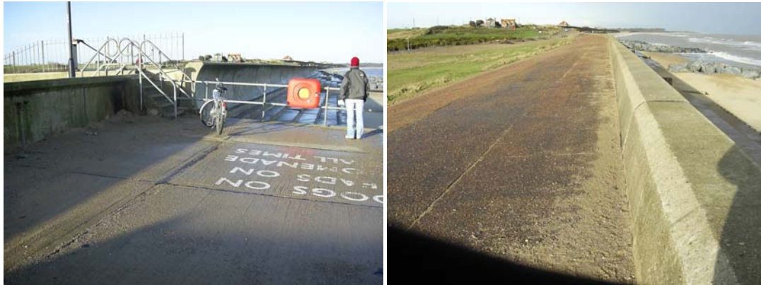
PLATE 4-5 SEA WALL NORTH OF SOUTHWOLD. THE SEA WALL IS PROVIDING COASTAL FLOODING PROTECTION.
