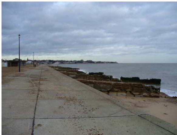
PLATE 4-10 EXAMPLES OF GROYNES AS COASTAL FLOOD DEFENCES IN FELIXSTOWE
