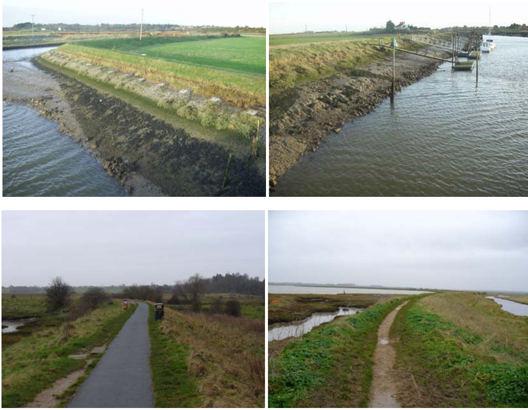
PLATE 4-1 EARTH EMBANKMENTS. THE EARTH EMBANKMENTS PROVIDE COASTAL PROTECTION BY RAISING THE LAND LEVEL OVER WHICH WATER HAS TO TRAVEL IN ORDER TO INUNDATE INLAND AREAS. THESE EMBANKMENTS CAN BE RE-ENFORCED AT THE BASE WITH CONCRETE. (SELECTION OF EARTH EMBANKMENTS IN SOUTHWOLD (TOP) AND WOODBRIDGE (BELOW)).
