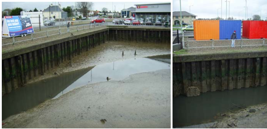
PLATE 4-6 SHEET PILE WALL IN LOWESTOFT AS AN EXAMPLE OF A FLOOD DEFENCE
