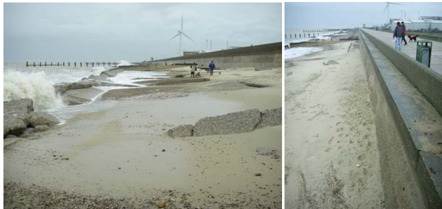
PLATE 4-3 SEA WALL. THE LOWESTOFT NORTH DENES SEA WALL IS PROVIDING COASTAL FLOODING PROTECTION (THE CONCRETE DEBRIS ON THE BEACH IS THE REMENENTS OF AN OLD COLLAPSED SEA WALL BUT MAY STILL PROVIDE SOME PROTECTION AGAINST SCOUR)
