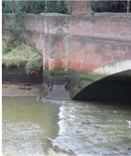
PLATE 4-11 EXAMPLE OF A WEIR AS A FLUVIAL FLOOD DEFENCE IN WOODBRIDGE
