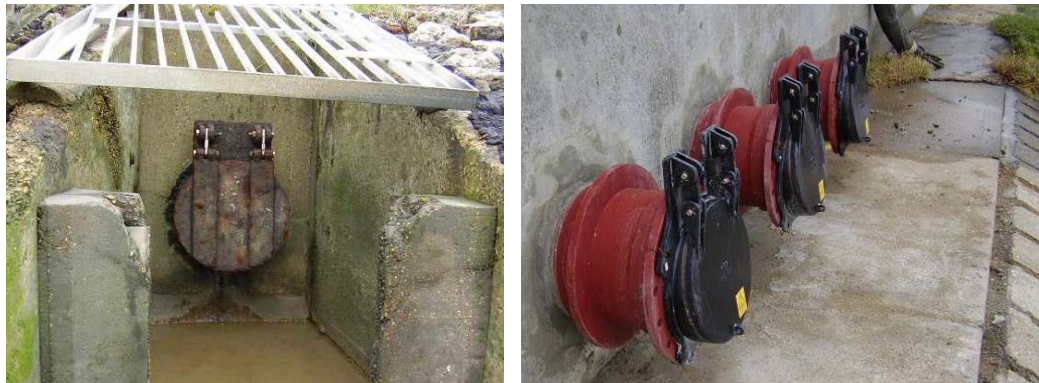
PLATE 4-8 EXAMPLES OF CULVERTS INSTALLED THROUGH FLOOD DEFENCES SHOWING TIDE FLAPPED OUTFALLS TO PREVENT A BACKWATER EFFECT DURING HIGH TIDE EVENTS.
