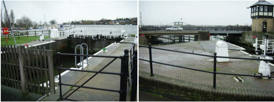
PLATE 4-9 EXAMPLES OF LOCK GATES IN LOWESTOFT AS FLOOD DEFENCE MECHANISMS.
