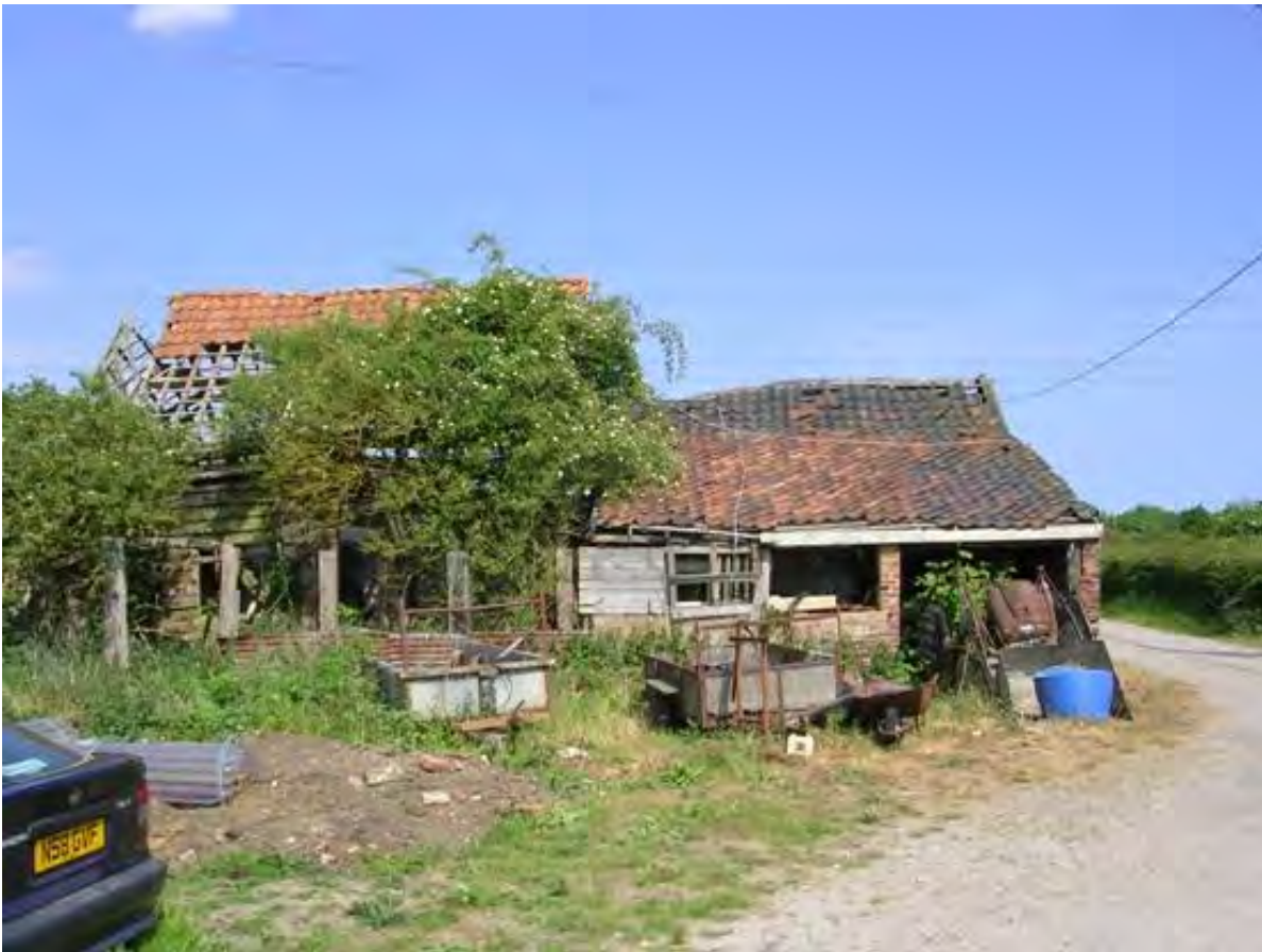
Picture 3: The barn viewed from the west (in front of the farmhouse). The building is in poor condition.
