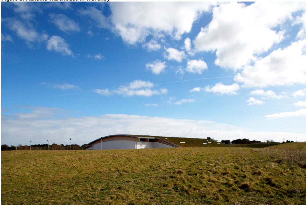
Figure 8: Adnams Warehouse in Waveney
