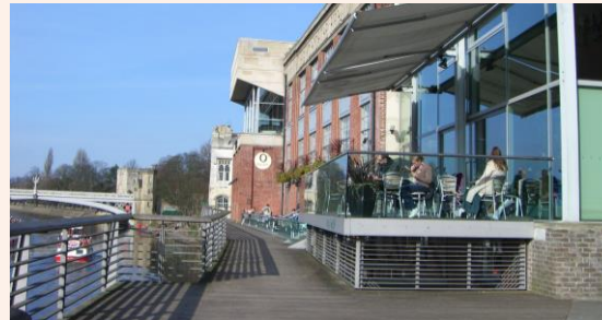
Above: Attractive waterfront development with a strong frontage, such as this example in York, should be encouraged in the Western End of Lake Lothing area.
